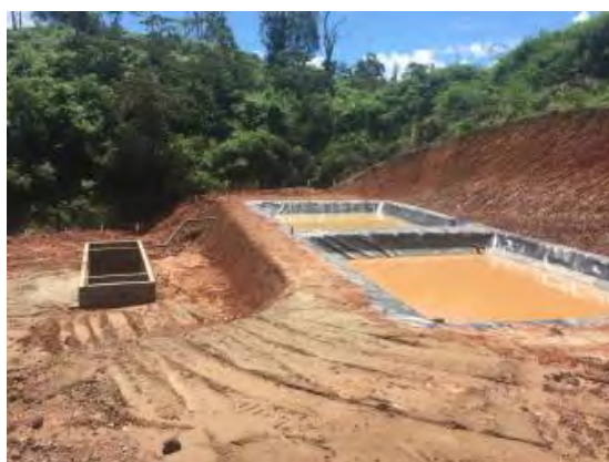
Photograph 17: Treatment ponds and Wetland Construction
