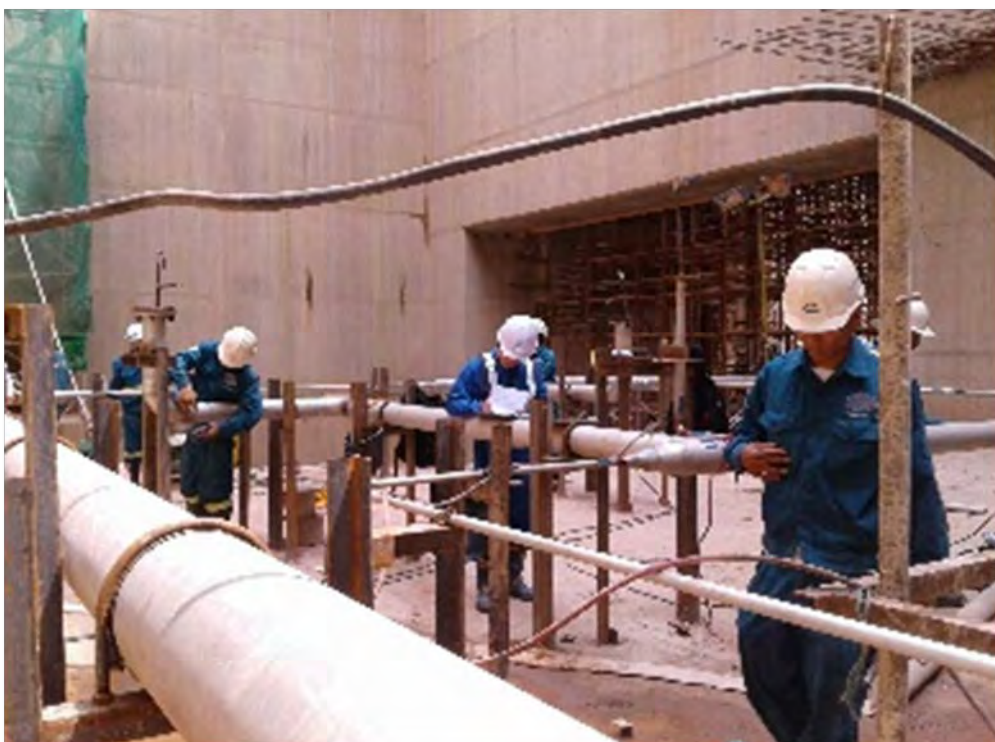
Photograph 1: Embedded piping installation (Main powerhouse)
