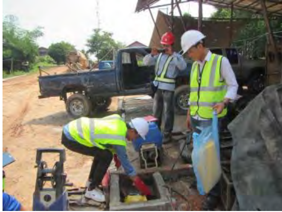
Photograph 8: Workplace hazardous waste management training for Loxley’s RCR sub-contractor (230 kV TL)
