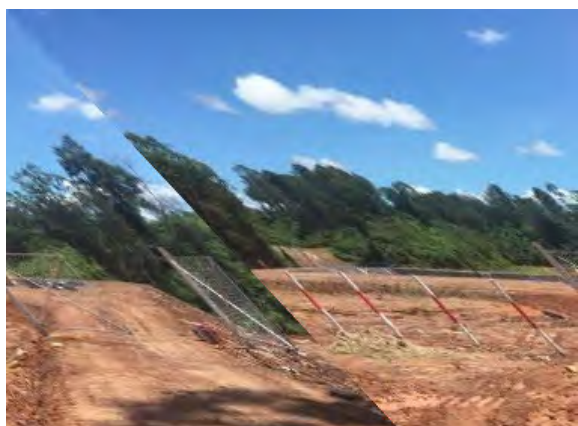
Photograph 16: Temporary fence and gate construction at HS Landfill
