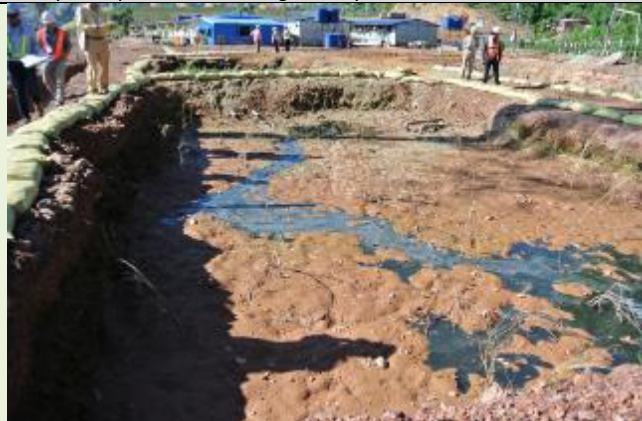
Photo shows improper construction of tank walls or berms. Collapsed berms at Song Da 2 Camp have contaminated stone and sand filters with mud balls. Mud and clay soil needs to be removed from the surface of the gravel filters; berms need to be lined with rip-rap or concrete
