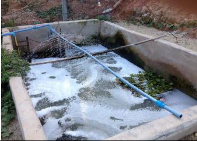
Combined wastewater "aeration" tank at Main Contractor's Camp. This tank is not adequate to be considered as an aeration tank; there is no separation of solids; wastewater is released to the environment before meeting effluent standards.
