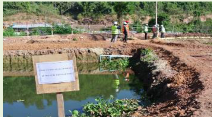
Photo shows improperly designed and built wastewater treatment pond. Shape and size of wetlands at Song Da 2 camp inappropriate; shape should be rectangular 3:1 L: W minimum, not square design. Aquatic plants need to follow specifications of Consultant for wetlands treatment. There is no chlorine contact tank or monitoring tank to check the quality of the treated effluent as specified by the Consultant.
