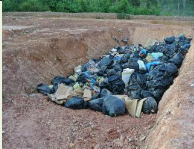
Above: Location of sanitary landfill for the NNP1 project to be built and operated by a private contractor supervised by the Owner. Pictures shows one "temporary pit" partially filled with construction and camp wastes. These wastes were not separated for recovering recyclable materials. The temporary pits will be emptied and re-constructed in a properly designed sanitary landfill. The pits will be lined with an impervious layer of compacted clay. A leachate collection system will be installed and connected to a series of leachate evaporation ponds. The NNP1 landfill site should also include a temporary storage facility for separation and storage of recyclable materials and hazardous wastes. NNP1 will manage the site for both and construction and operation phases.
