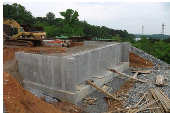
Plate 2-6: Example of the proposed Bridge Abutment
