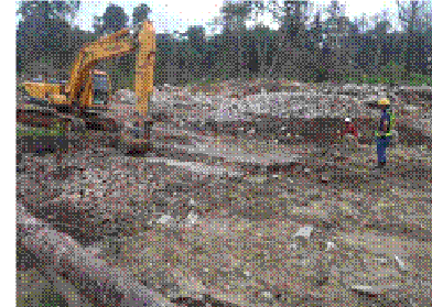
Km 16+00 Quarry Settlement pond installation
