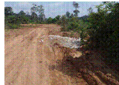
Sta. 17+200_Drainage improvement by gravel filling
