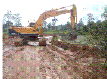
Sta. 17+200_Drainage improvement by gravel filling
