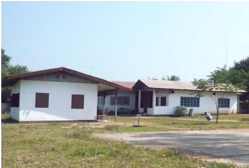
Figure 3.10 Bolikhan district hospital
