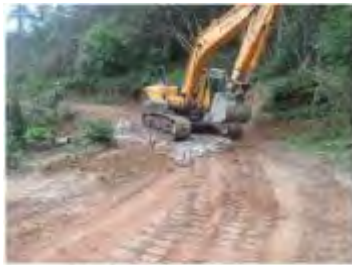
Sta. 15+200 Road improvement by Gravel filling
