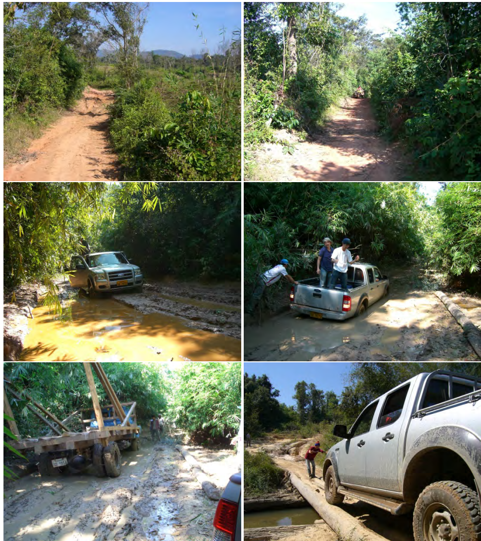
Figure 3.6 The existing access road
