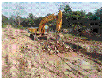
Sta. 22+200 Road improvement by gravel filling
