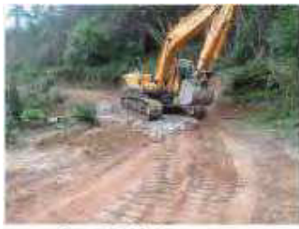
Sta. 15+200 Road improvement by Gravel filling
