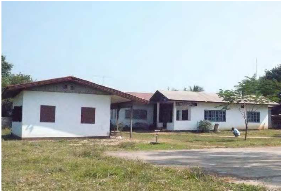
Figure 3.10 Bolikhan district hospital
