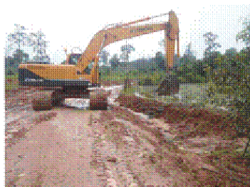
Sta. 17+200_Drainage improvement by gravel filling
