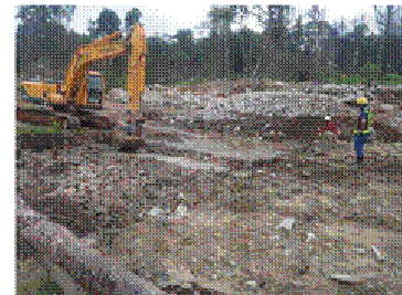
Km 16+00 Quarry Settlement pond installation
