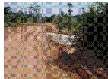
Sta. 17+200_Drainage improvement by gravel filling
