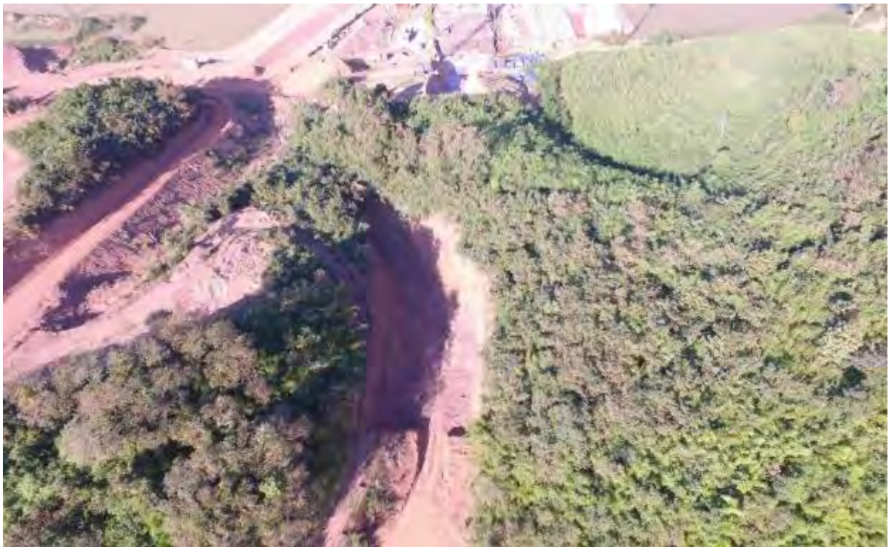
FIGURE 5-10 INTAKE MOUTH CANAL CONSTRUCTION AS OF 29 DECEMBER 2016
