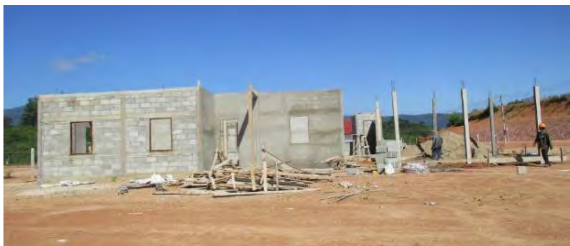
FIGURE 5-6 CONSTRUCTION OF HOUSE NUMBER 24 IN THE HSRA FOR HATSAYKHAM AS OF 28 NOVEMBER 2016
