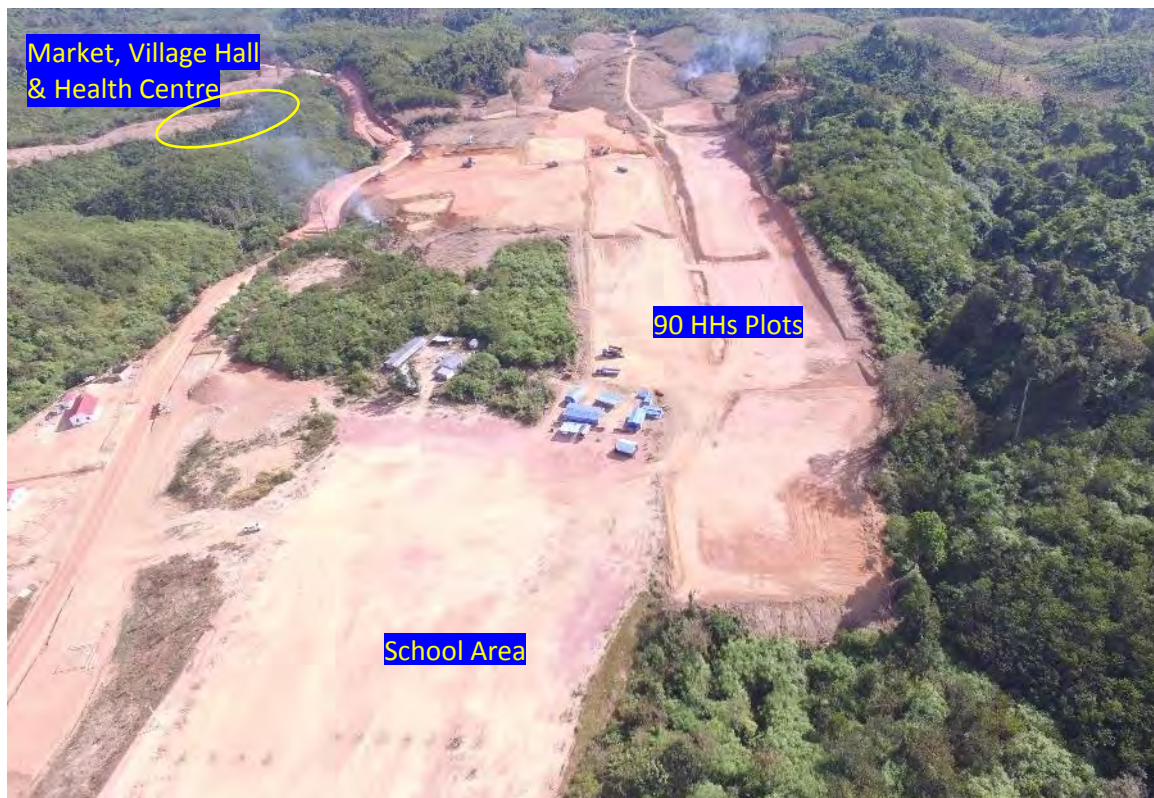
FIGURE 5-7 CONSTRUCTION PROGRESS OF LAND LEVELLING FOR 90 HOUSEHOLD PLOTS IN THE HSRA FOR 2LR AS OF 29 DECEMBER 2016
