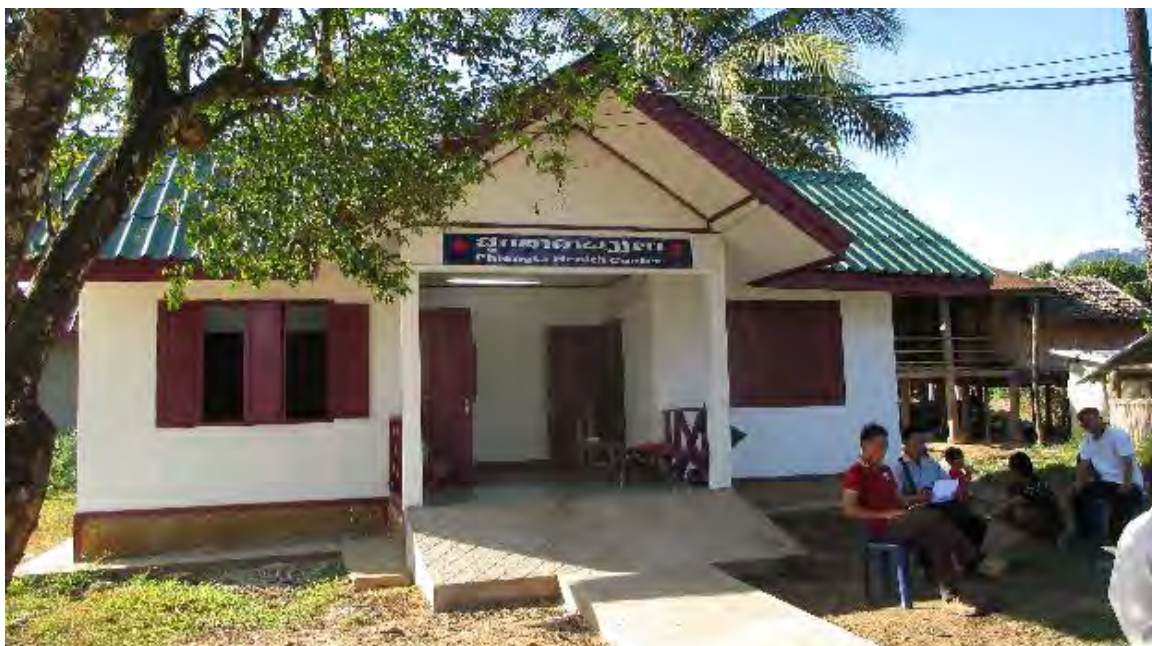
FIGURE 5-12 FINAL INSPECTION OF THE HEALTH CENTRE RENOVATION 28 NOVEMBER 2016
