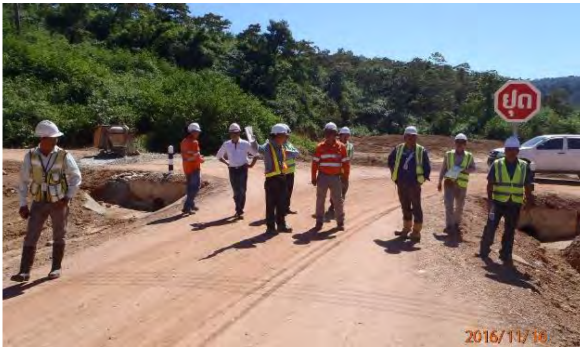
FIGURE 5-5 FINAL INSPECTION OF INTERNAL ROAD 16 NOVEMBER 2016
