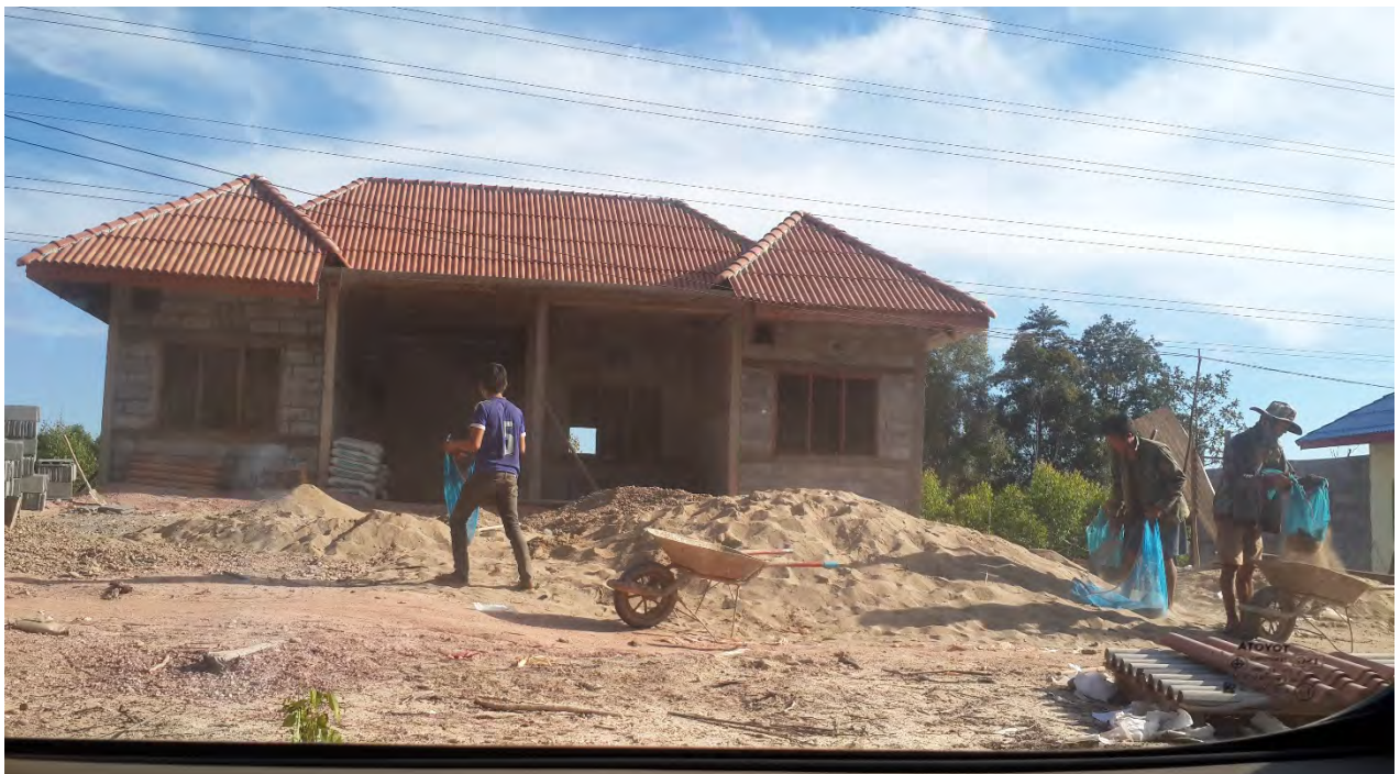
FIGURE 8-2 ONGOING CONSTRUCTION OF THEIR HOUSE BY A SELF-RESETTLERS FAMILY MOVING TO NONSOMBOUN VILLAGE (DECEMBER 2016)
