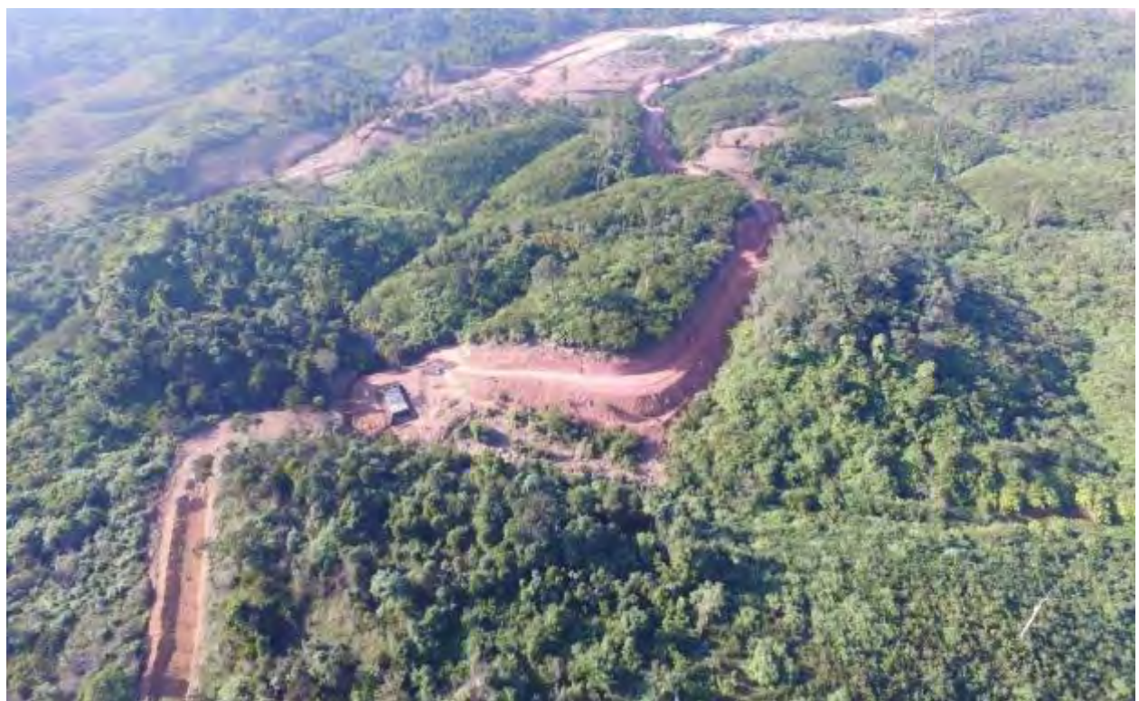
FIGURE 5-8 MAIN ROAD CONSTRUCTION 1.375 KM AS OF 29 DECEMBER 2016
