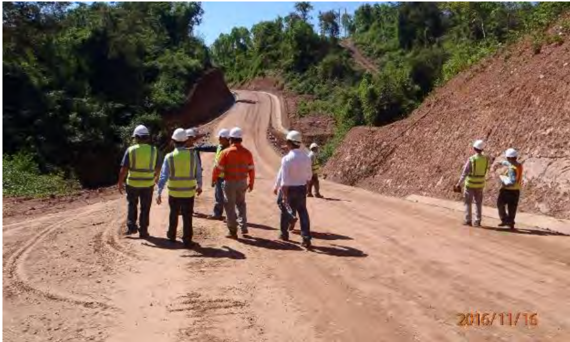
FIGURE 5-4 FINAL INSPECTION OF MAIN ROAD 16 NOVEMBER 2016
