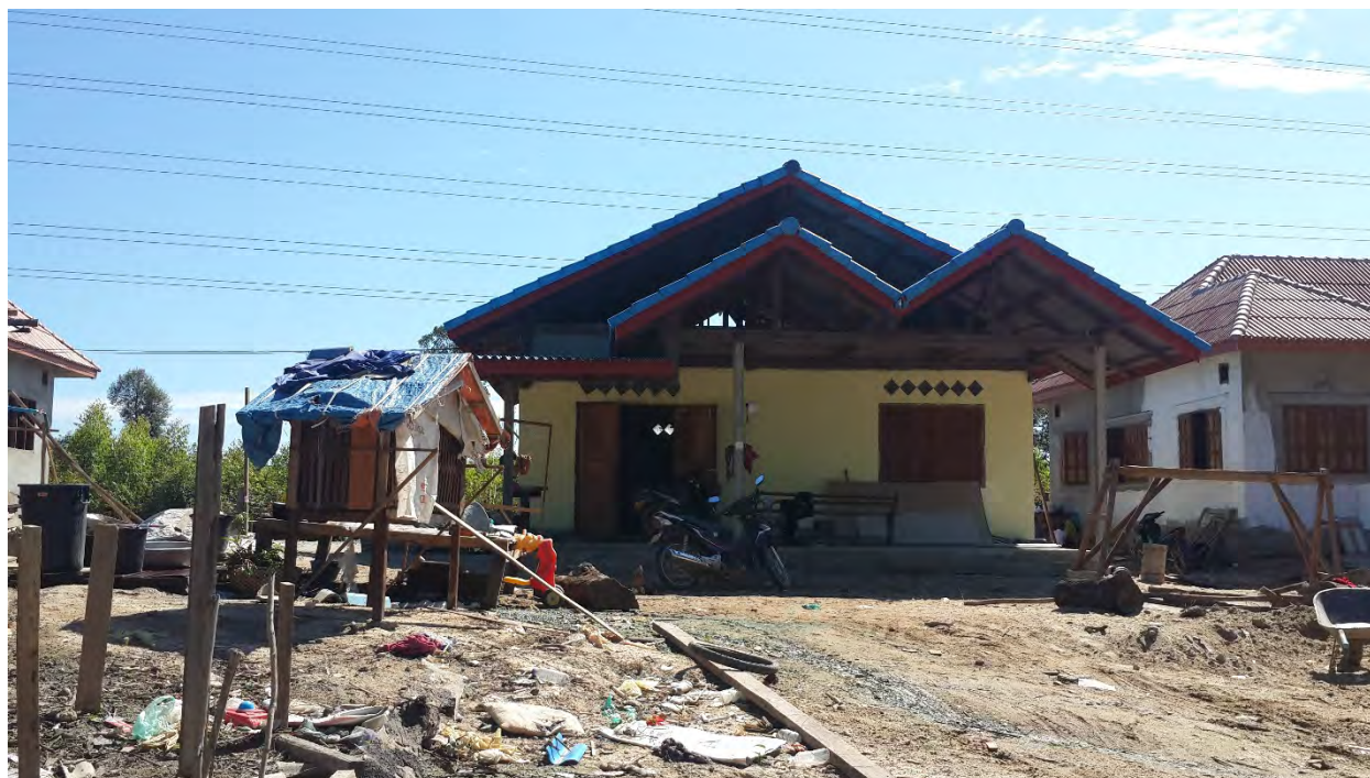
FIGURE 8-3 ONGOING CONSTRUCTION OF THEIR HOUSE BY A SELF-RESETTLERS FAMILY MOVING TO NONSOMBOUN VILLAGE (DECEMBER 2016)
