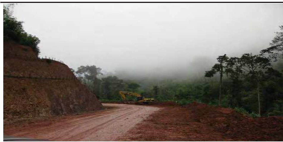
Figure 6.3 Large Sediment Load due to Unpaved Road
