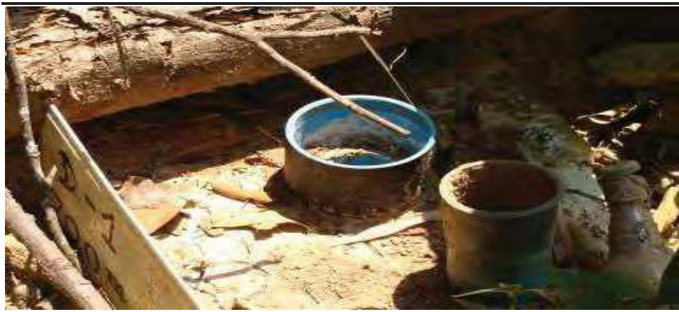
Figure 5.18 Stake Marking the Dam Site
