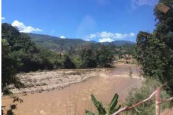
River section between main dam and re-regulation dam contains significant in-channel deposits and features
