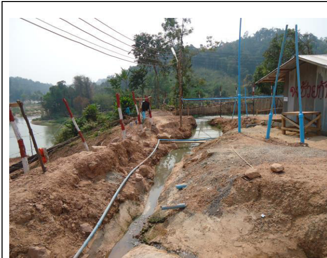
Photo 9 Right Tunnel grey water treatment pond
