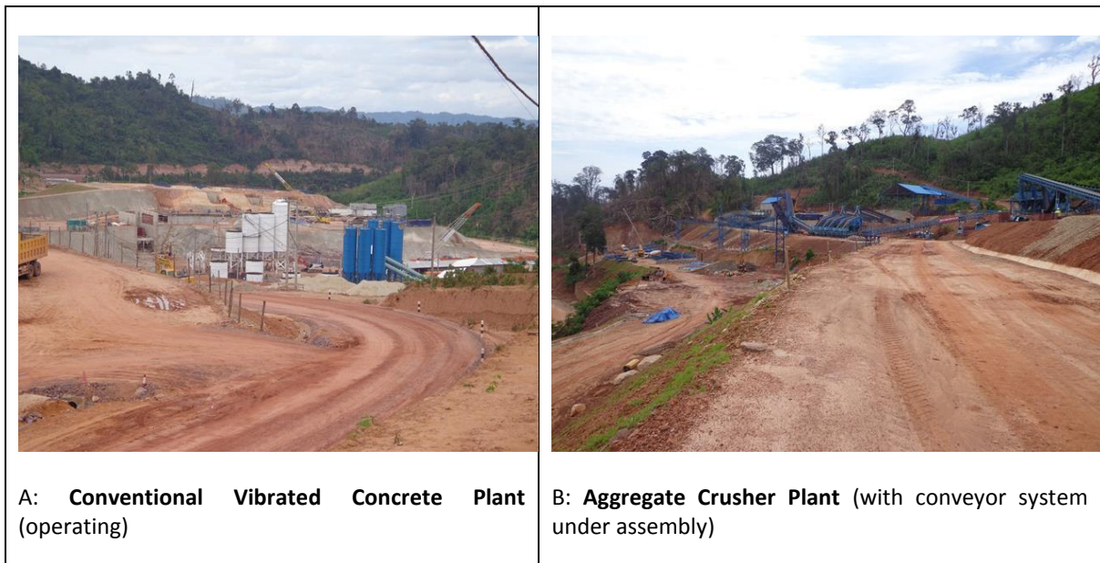
Photo 7 Construction related facilities
