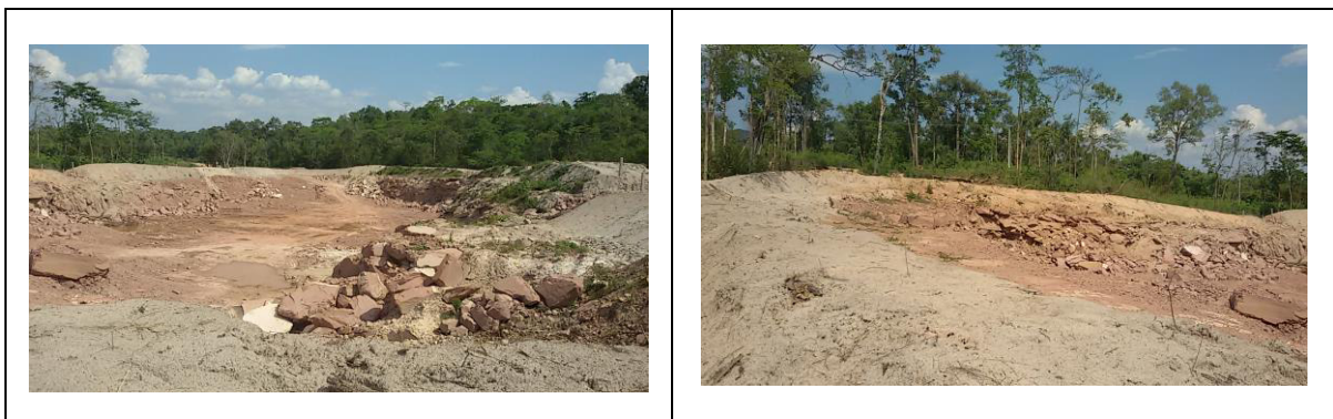
Photo 1 Main Access Road Quarry at STA9+400 – on standby
