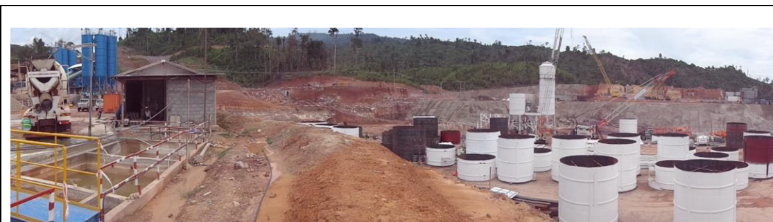
C: Roller Compacted Concrete plant (to right of photo, under construction).
