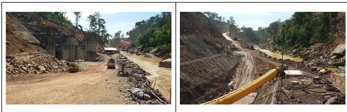
Photo 3 Diversion Tunnel Inlet head works (left photo looking downstream) and Outlet excavations (looking downstream), April 2015
