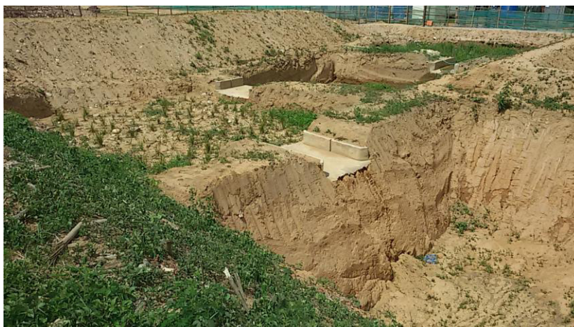
Photo 12 TCM Camp WWTS upgrade
