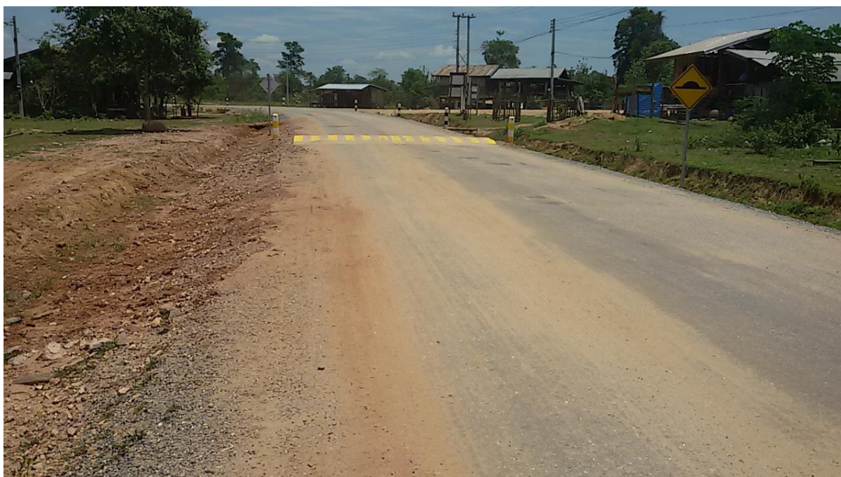
Photo 15 sealed road surface and speed bumps at Ban Hat Gnuin (April 2015).
