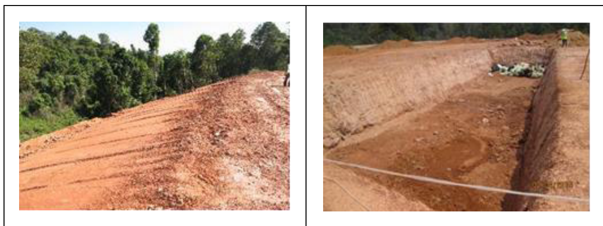
Photo 8 NNP1 landfill embankment works and one of the temporary pits (January 2015)
