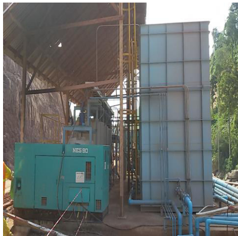
Photo 14 The effluent filtration system used at the tunnel outlet excavation site.
