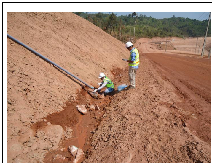
Photo 11 Sinohydro grey water treatment system discharge location
