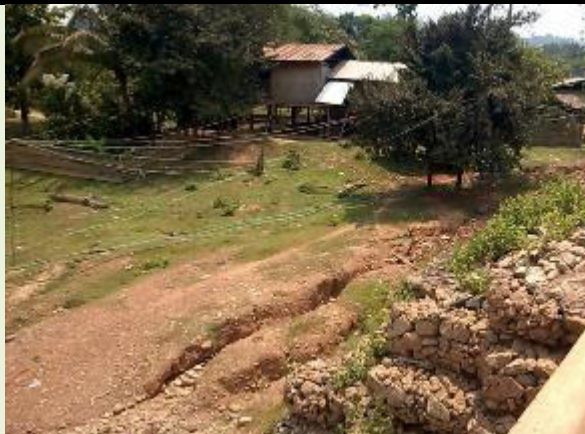
Erosion at the bridge on the Dam Access Road at Ban Thaheua , Zone 3
