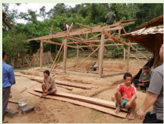
New buildings continue to be in Ban Sopyouak , Zone 2LR even after PAP have been informed of the official cut-off-date and asset surveys have been completed
