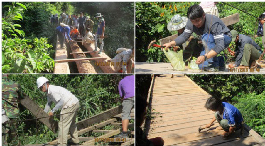
Repairing of suspension bridges at Sopyouak village, 19 November 2015
