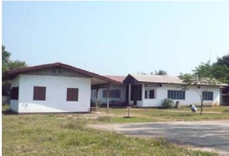
Figure 26 Bolikhan district hospital
