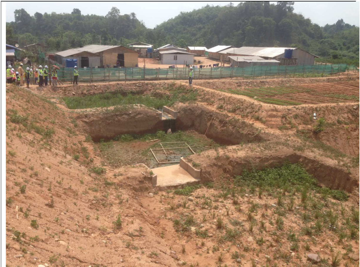
Waste water wetland filtration treatment system in TCM camp.
