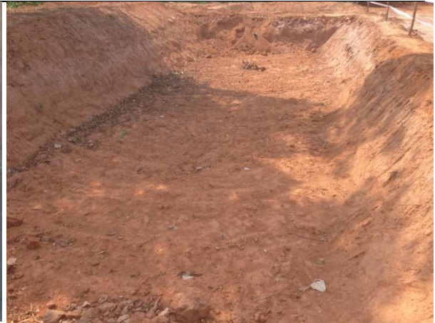
Preparing the waste water wetland filtration treatment system in the SongDa camp.
