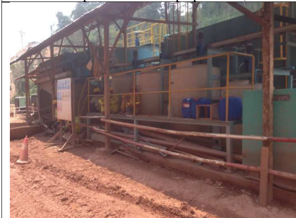
Waste water treatment plant of the water coming out from the tunnel excavation
