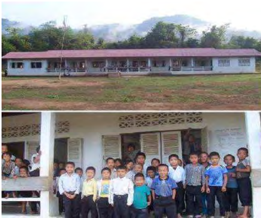
Primary school in Ban Sopyouak
