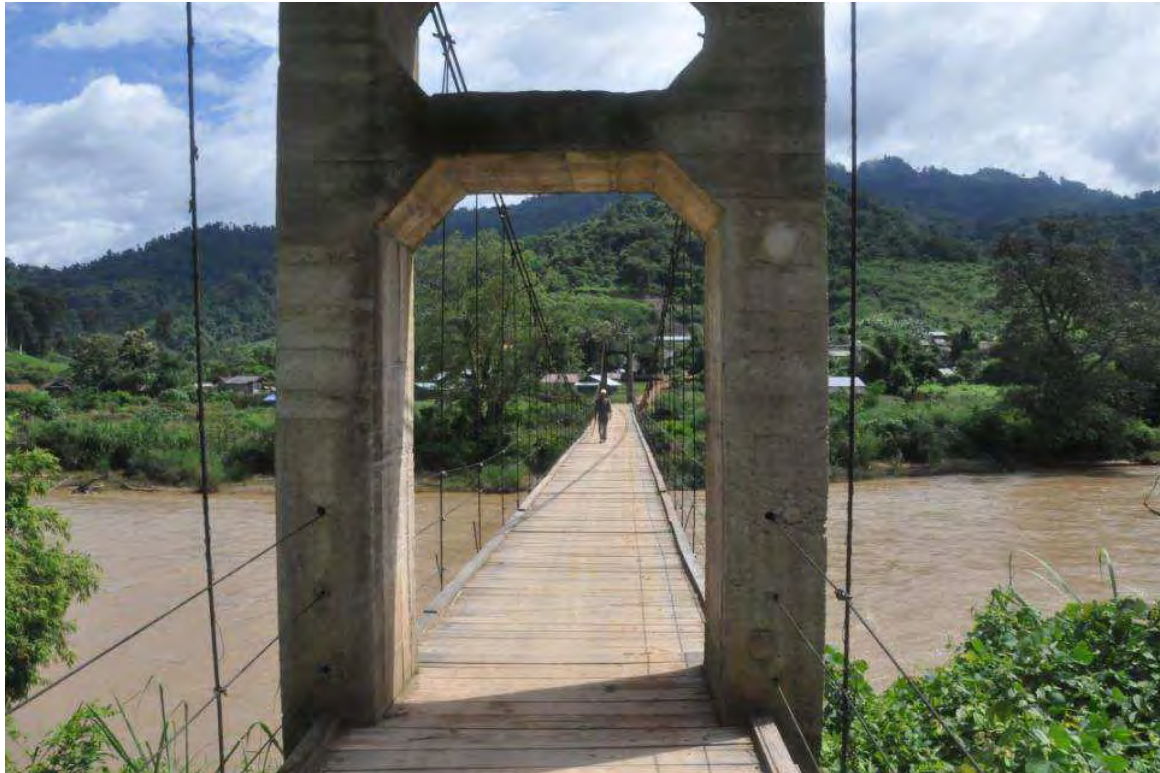
Figure 76: Suspension bridge across the Nam Ngiep
