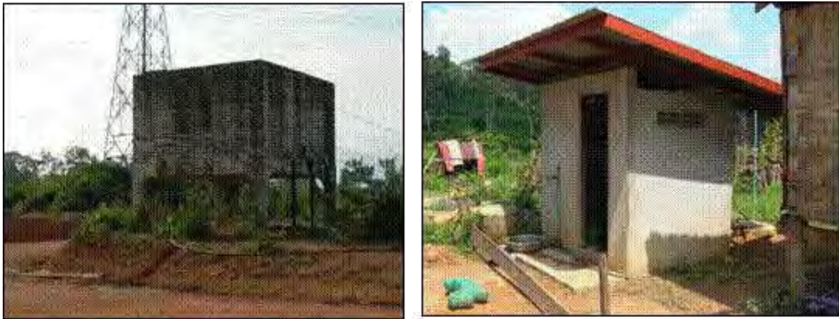
Figure 46: Water tank and tap water at Theun Hinboun Ex HPP
