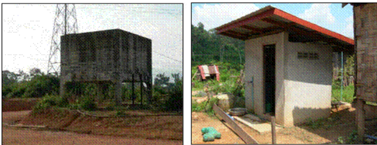
Figure 28 Example of water tank and tap water supply at Theun Hinboun Ex HPP
