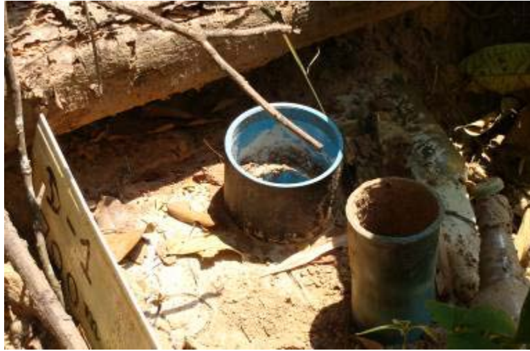
Figure 5-10 Stake marking the dam site.
