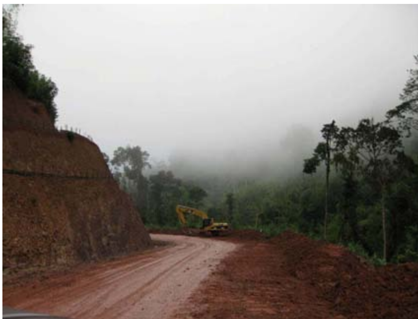
Figure 7-3 Large sediment load due to unpaved road.
