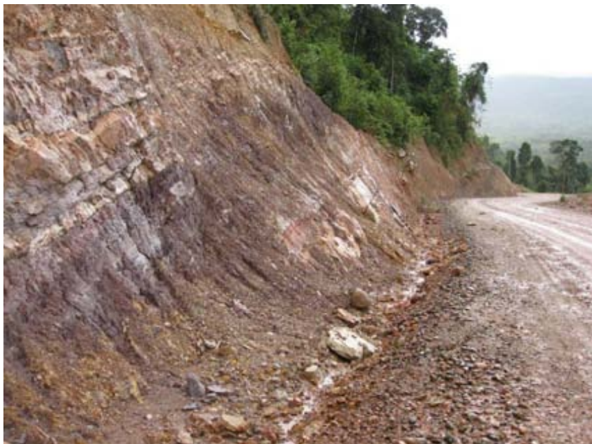
Figure 7-2 Water drainage channel provided along an elevated unpaved road.
