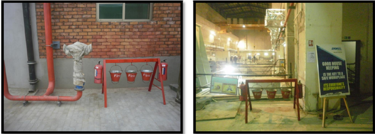
Photographs shows the Fire stand at different locations
