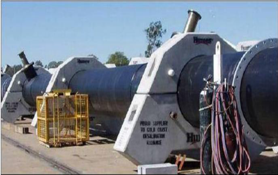
Figure 3: Waste water discharge system from the SWRO Plant.
