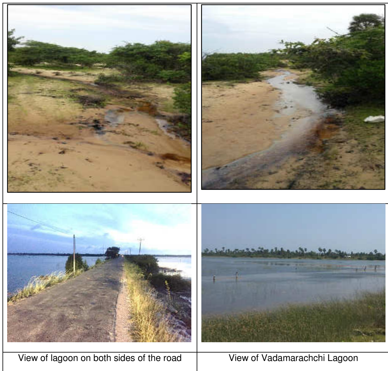
Photo 15: Drainage from the project site, December 2015
