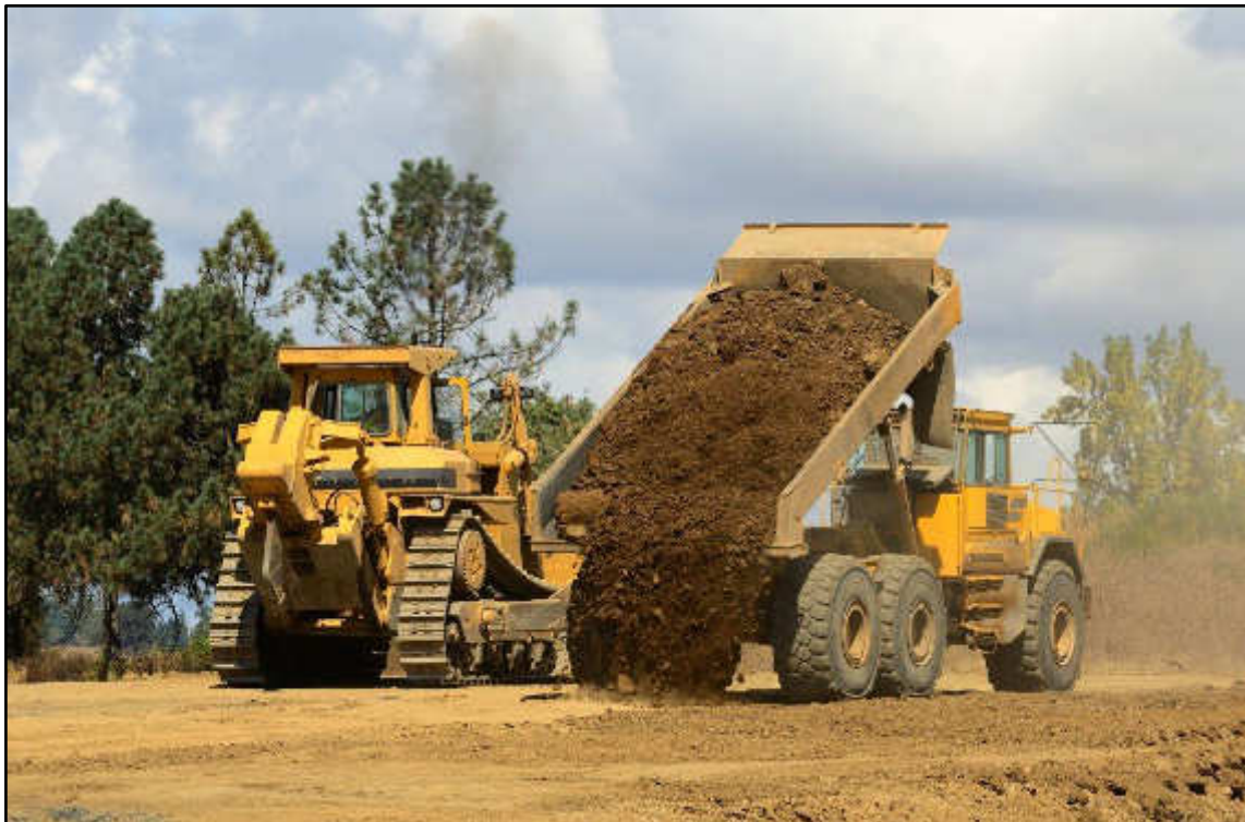
Photo 5: Bulldozer and dump truck conducting earthworks
