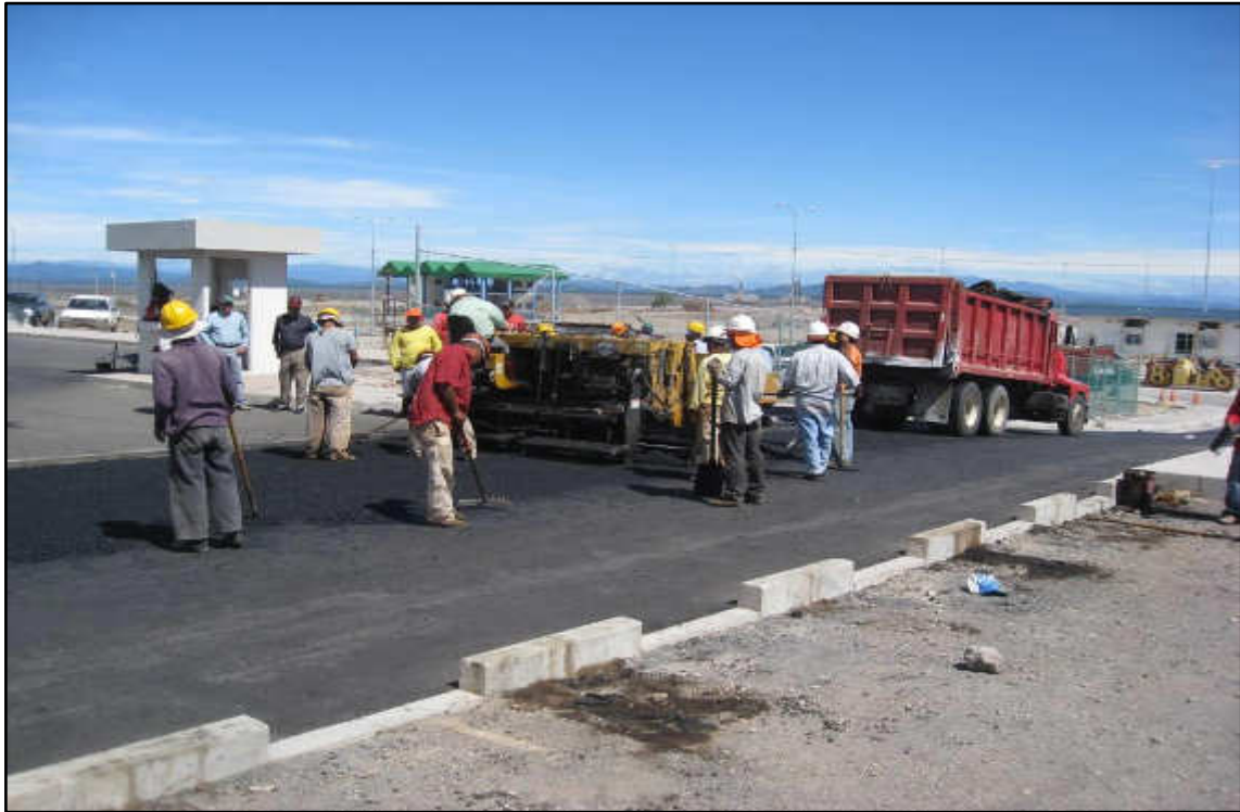
Photo 4: Applying a bitumen top coat to a new construction site access road
