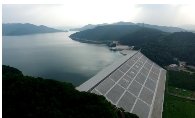
Figure V-7 Reconstructed downstream slope protection for Tanghe Reservoir dam
