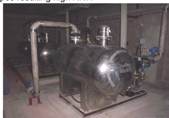
Figure IV-3+4 rusty Pumping Equipment
