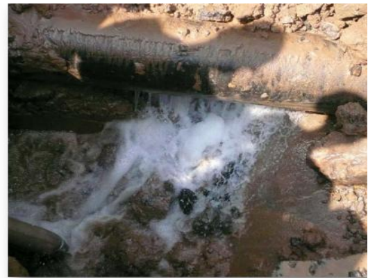
Figure IV-1+2 Aged pipes resulting high NRW
