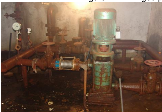
Figure IV-3+4 rusty Pumping Equipment
