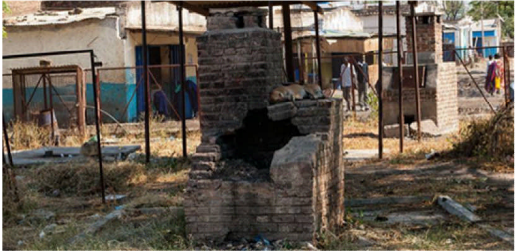
Figure 2-2: Old Medical Waste Incinerator, Malakal
