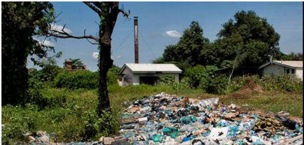
Figure 3-5: Incinerator of the Juba Teaching Hospital
