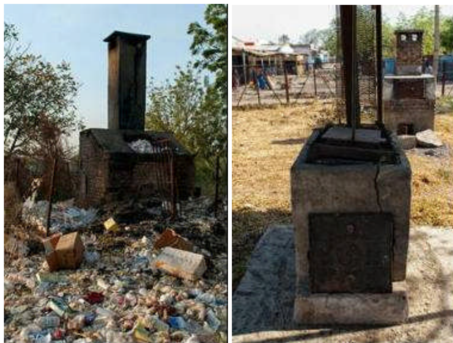
Figure 6-17: Old and broken incinerators, Malakal
