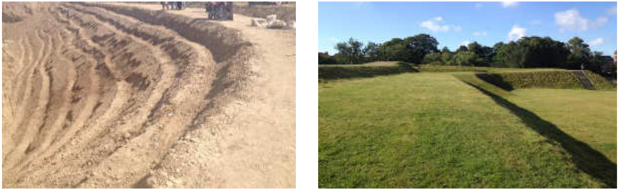
Figure: Example of muck benching and re-vegetation.
