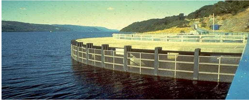
Figure: Example of fish screens at hydropower intakes.
