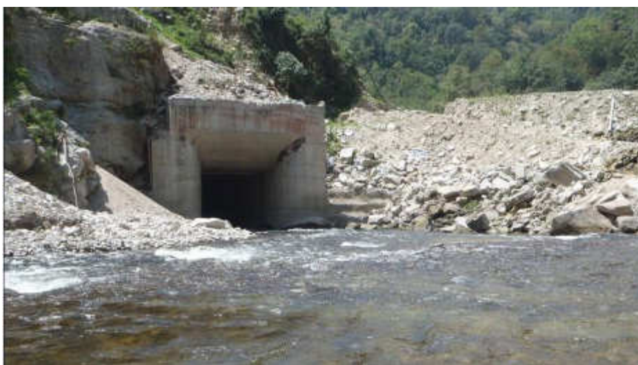
Figure 2-5: Typical cofferdam and diversion tunnel (at Dagachhu).
