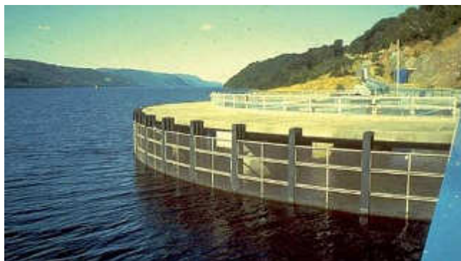
Figure 6-13: Example of fish screens at hydropower intakes.
