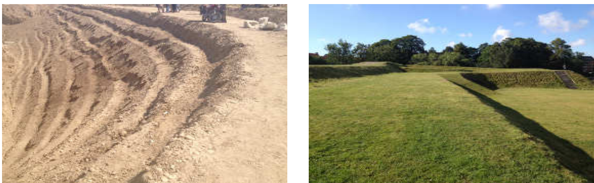
Figure: Example of muck benching and re-vegetation.
