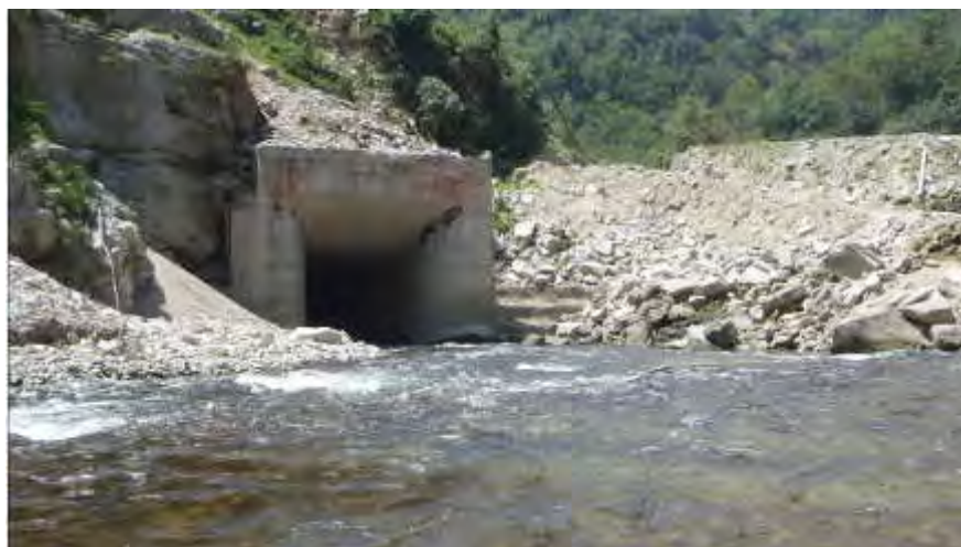
Figure 2-5: Typical cofferdam and diversion tunnel (at Dagachhu).
