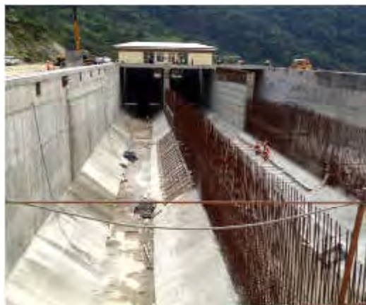
Figure 2-6: De-silting facility under construction at Dagachhu.
