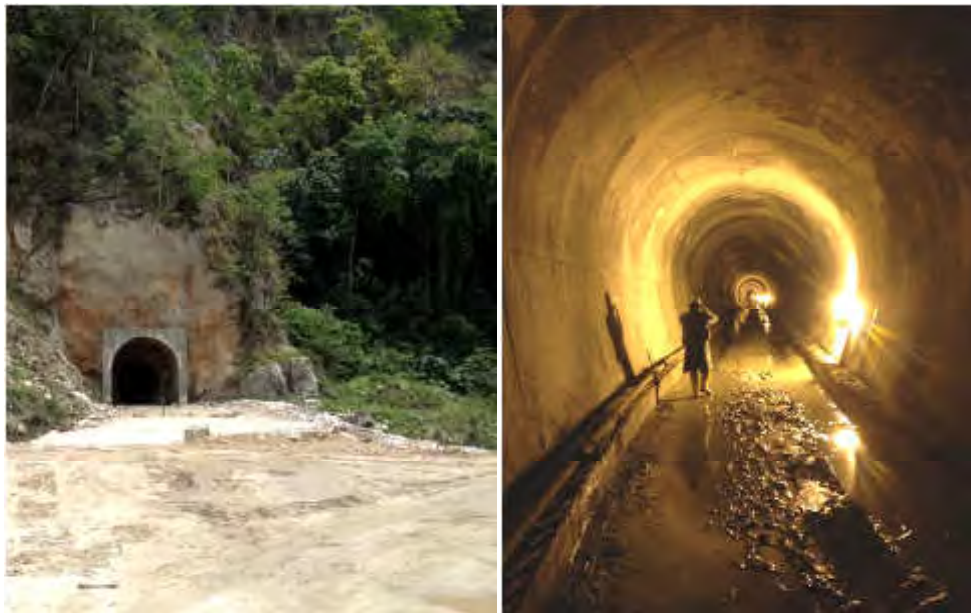
Figure 2-7: Head race tunnel at Dagachhu.
