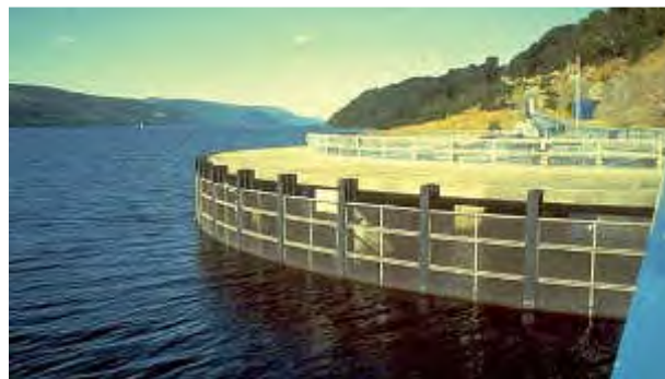
Figure 6-13: Example of fish screens at hydropower intakes.
