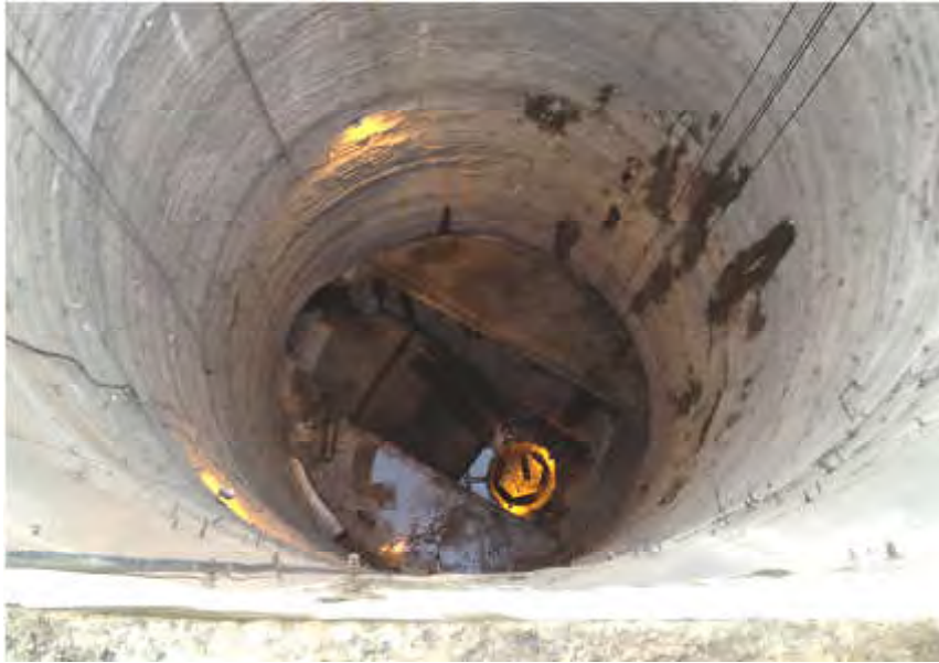
Figure 2-8: The surge shaft under construction at the Dagachhu site.
