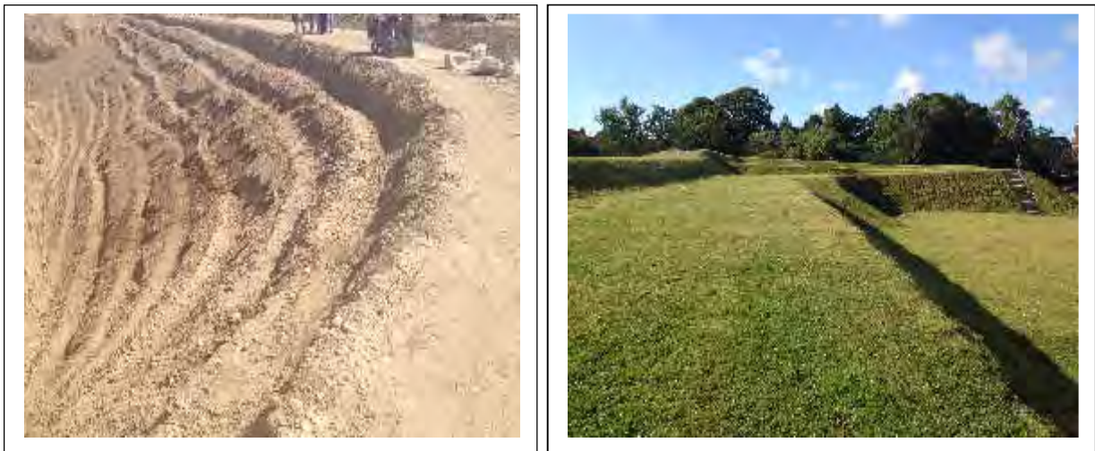
Figure 6-9: Example of muck benching and re-vegetation.
