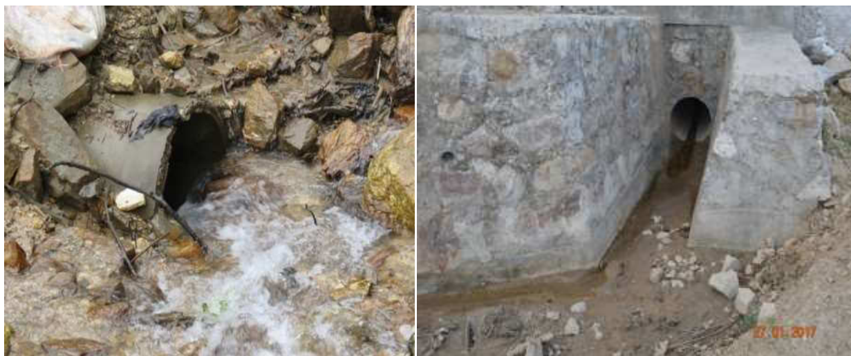
Figure 13.1 Hume pipes, and drains to divert streams along access roads
