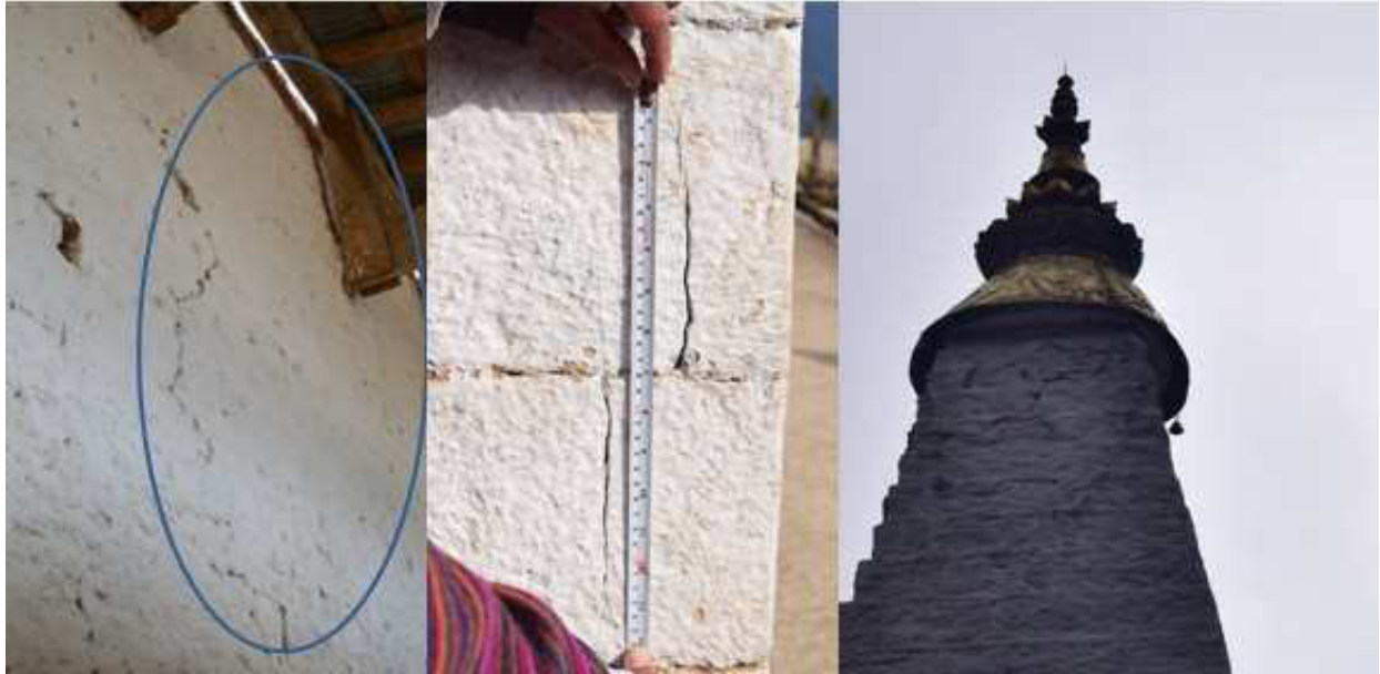
Figure 34.1 Crack mapping of structures at five locations
