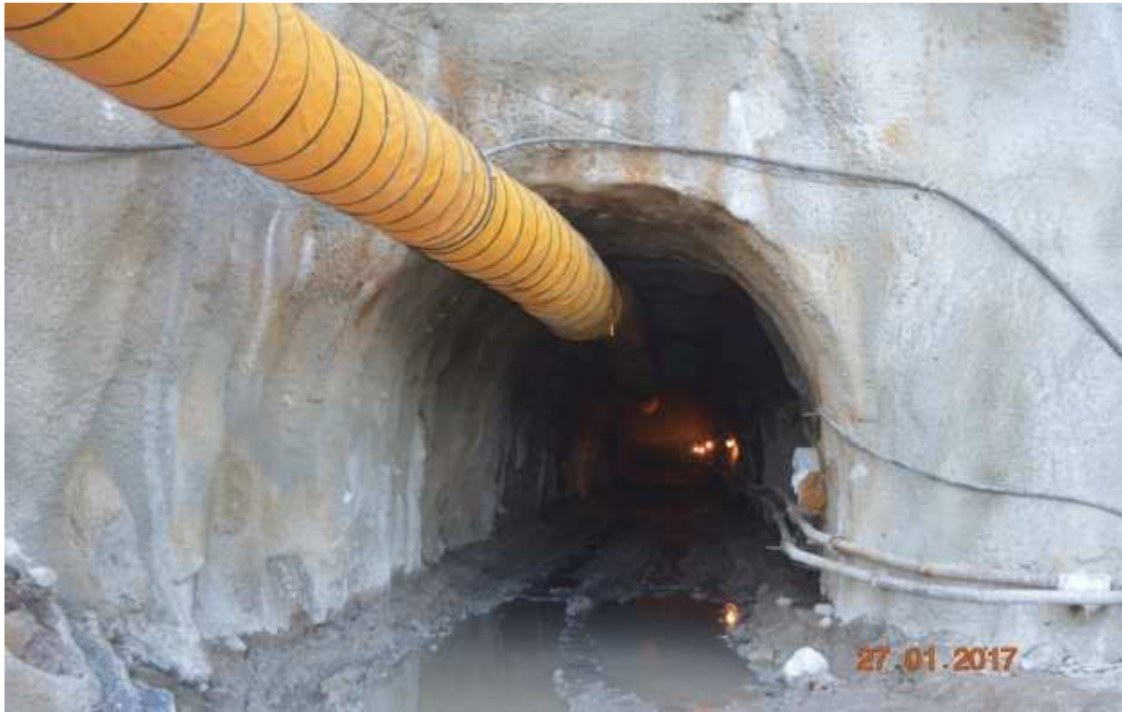
Figure 30.1 Ventilation system and illumination
