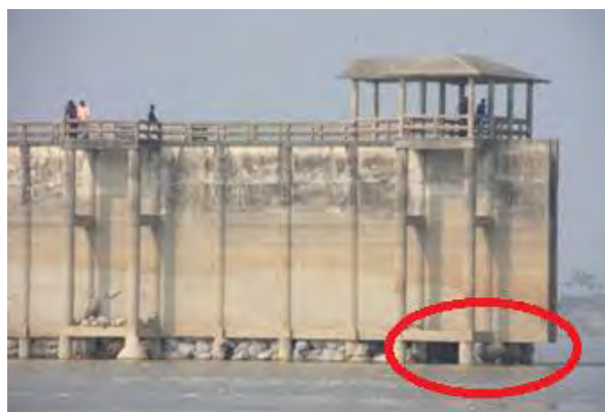
Figure A4.6: Erosion Damage Upstream of Enayetpur, Post-2012
