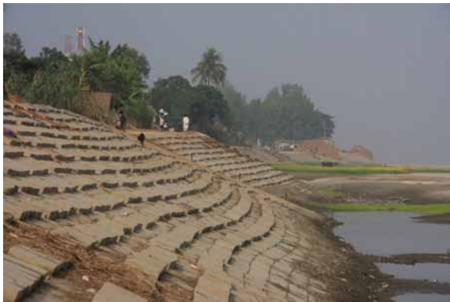
Riverbank Protection alongside JRB-1
