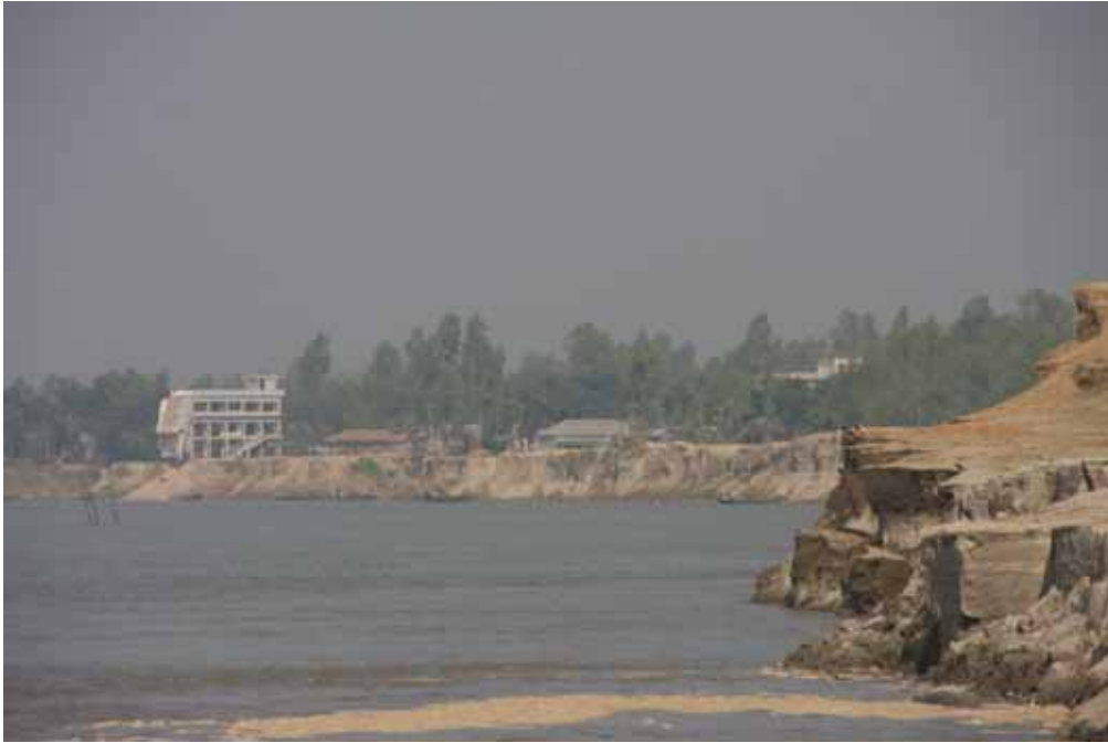
Unprotected riverbank at PLB-1, Harirampur area
