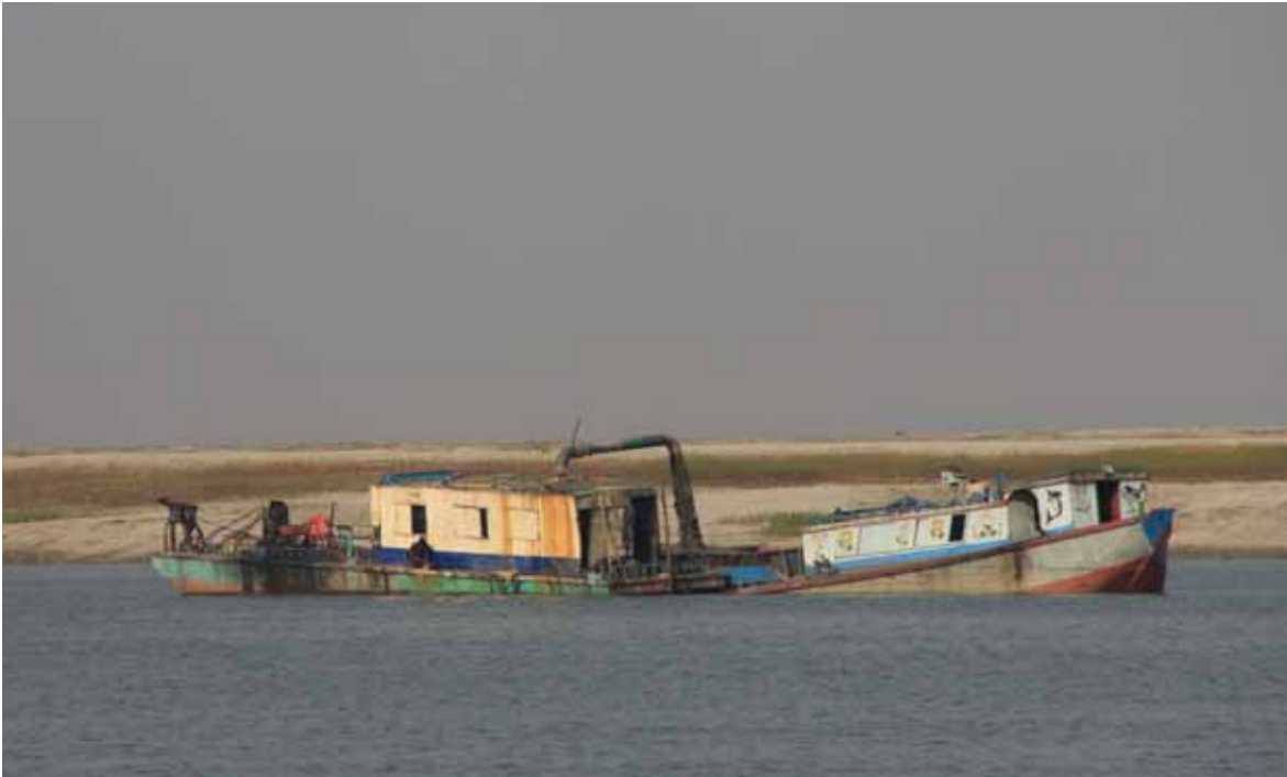
Dredging of sand for embankment construction
