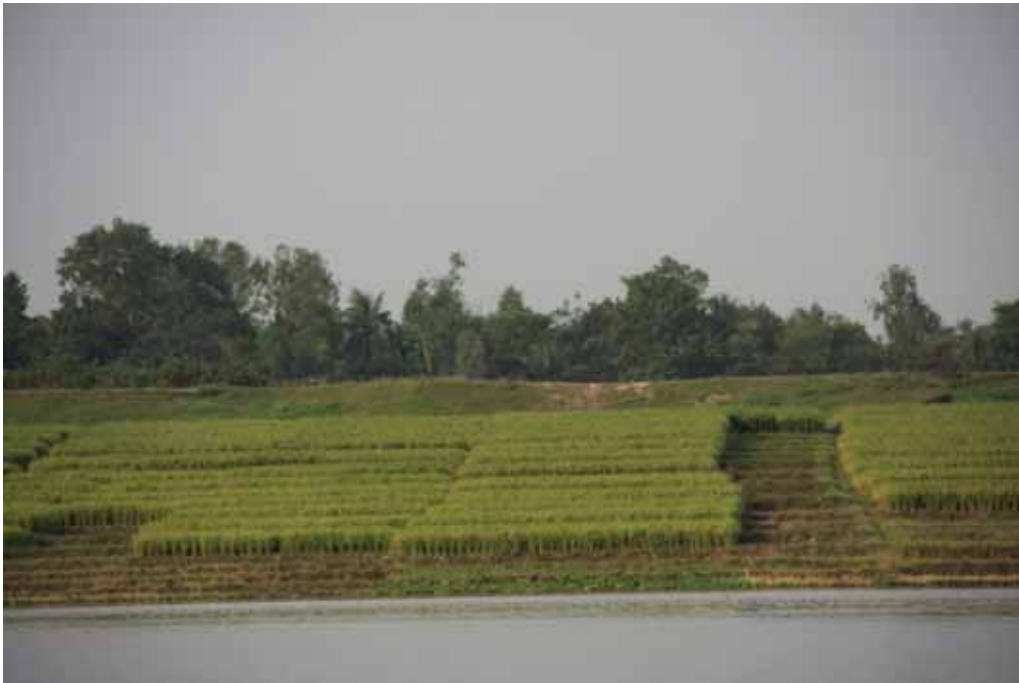
Embankment along the Hurasagar/Baral
