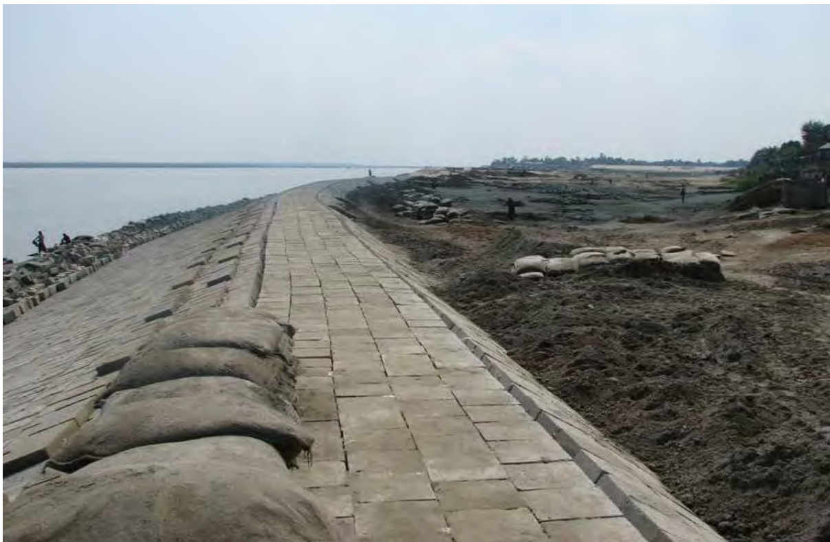
Figure 2-28: Photograph an Embankment Newly Re-Constructed with Cement Blocks
