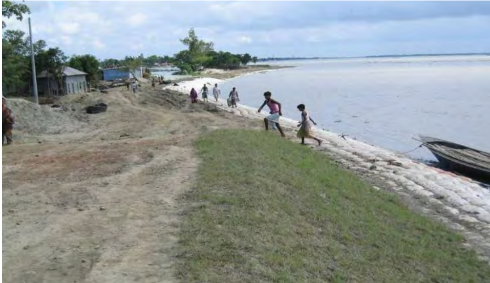
Figure 2-27: Photograph of an Old Earthen Embankment after HHs were Resettled and the Final (Underwater) Protection was completed
