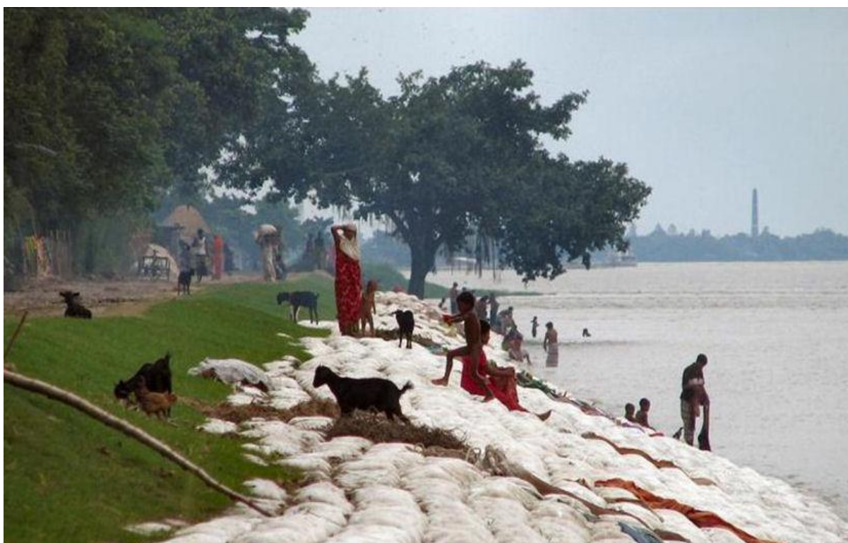
Figure 2-30: Photograph of Re-Constructed Embankment Finished Permanent Protection with Grout Filled Mattress
