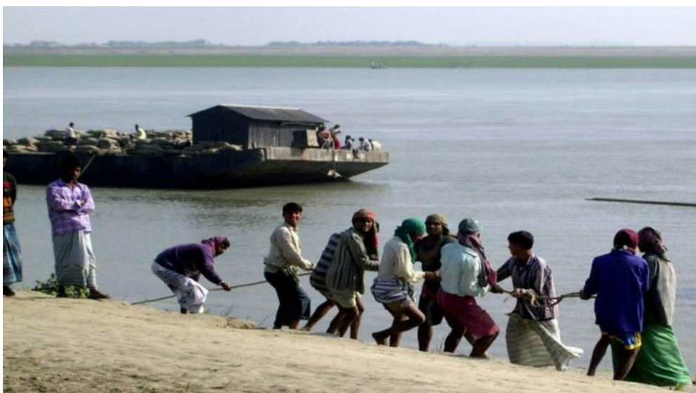
Figure 2-26: Photograph of Pulling Geobag Dumping Barge to a new Location
