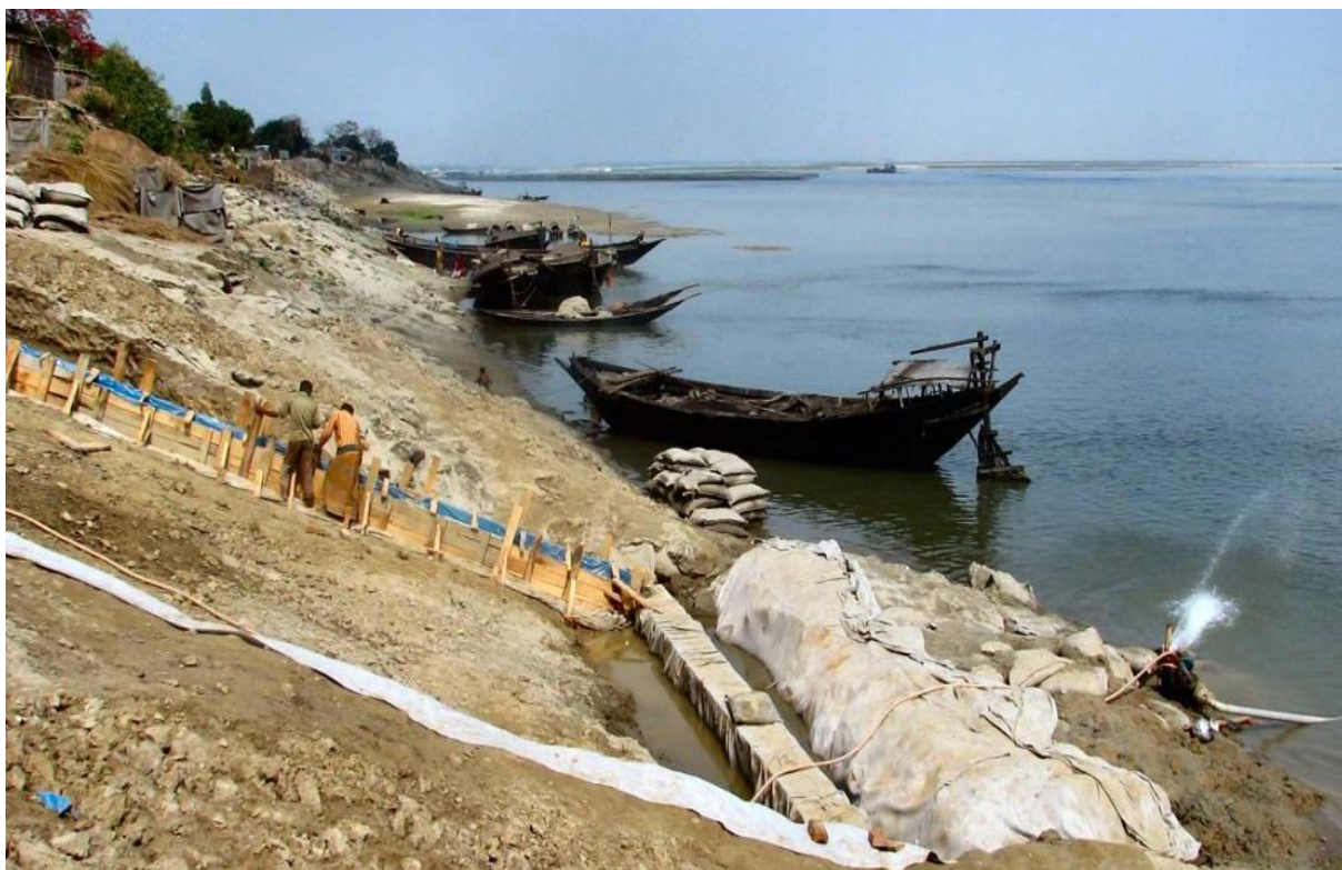
Figure 2-29: Photograph the old Embankment Preparing for Permanent Protection with Grout Filled Mattress
