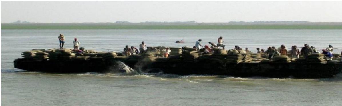
Figure 2-25: Photograph of Primary Protection through Systematically Dumped Geobags from Barge
