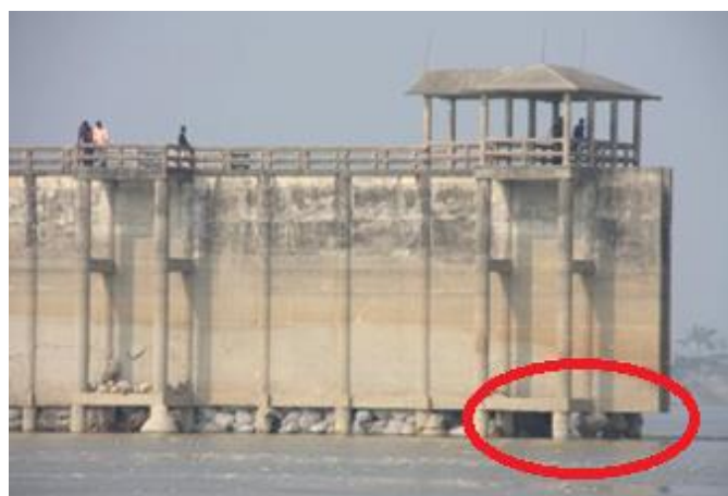
Figure A7.6: Erosion Damage Upstream of Enayetpur, Post-2012
