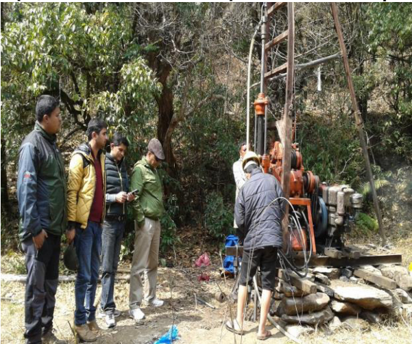
Drilling Works for Soil Investigation by the Contractor
