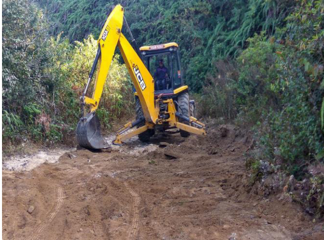
Access Road Maintenance and Upgrading by the Contractor
