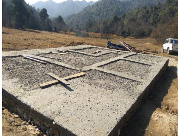
Site Camp Location with Completed Foundation
