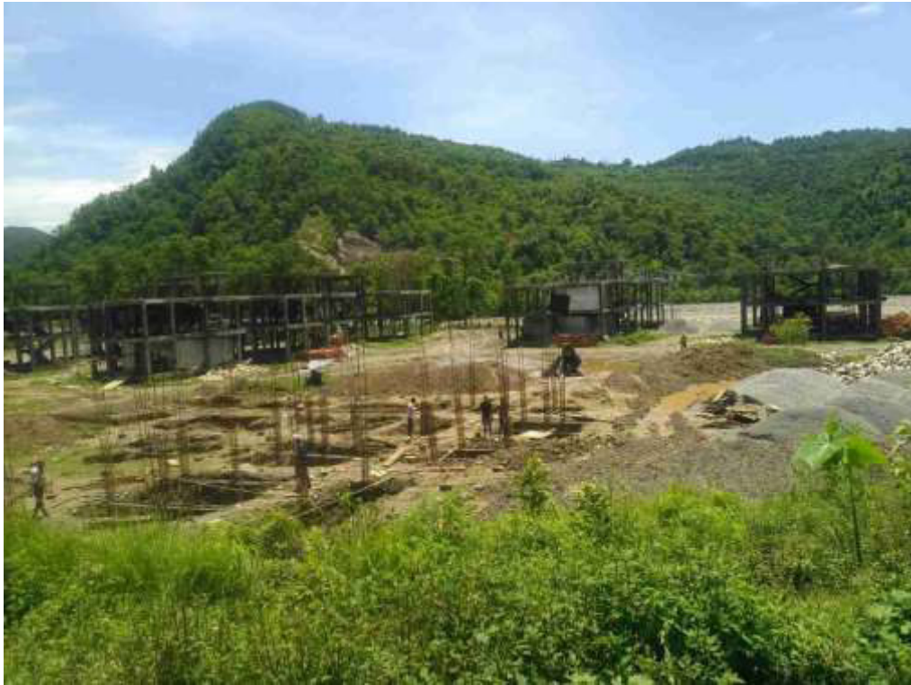
Figure 3: Construction of Camp Facilities
