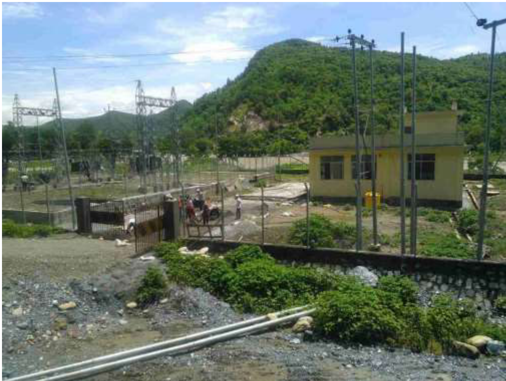
Figure 4: Construction of Sub-station
