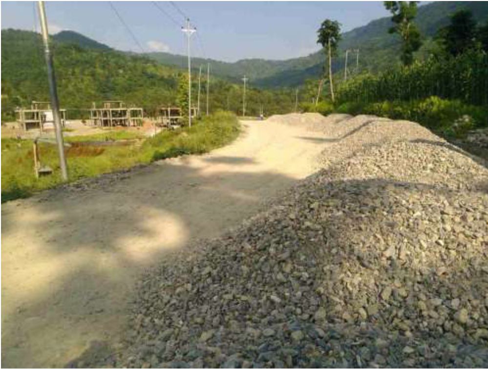
Figure 5: Access Road Construction
