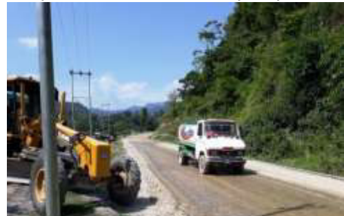
Progress of access Road from Chapaghat to Dam Site
