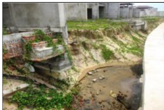
DIRECT DAMAGES OF EROSION
