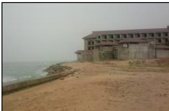
RESORT CONSTRUCTION ABANDONNED DUE TO EROSION RISK
