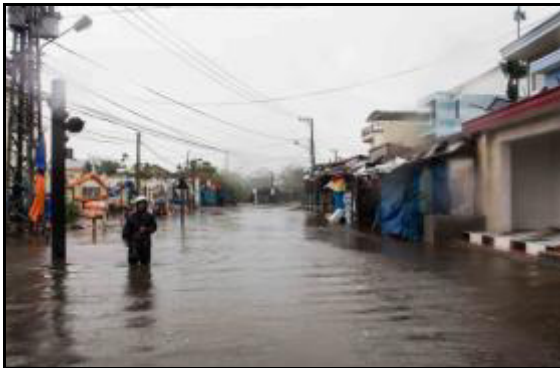
FLOODING OF LOW LYING AREAS IN THE CITY
