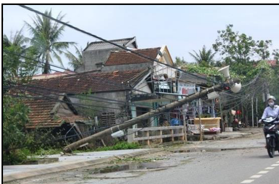
ELECTRIC AND TELEPHON LINES
