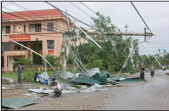
ELECTRIC POLES BROKEN
