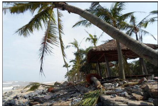
SUN SPA RESORT, AT THE TIP OF BAO NINH WAS SERIOUSLY DAMAGED BY WUTIP
