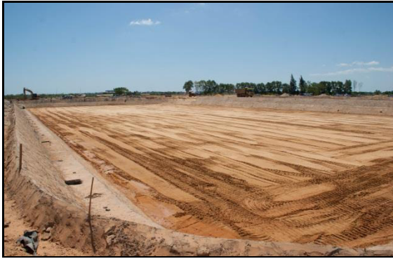
ONE OF THE FACULTATIVE POND UNDER CONSTRUCTION
