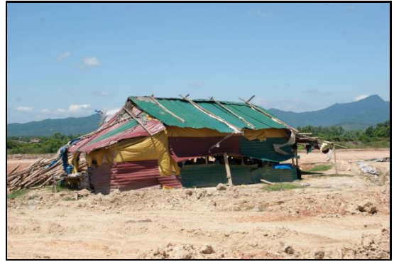
VERY POOR STANDARD FOR WORKER'S BUILDING INCLUDING KITCHEN
