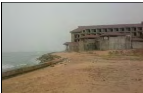
RESORT CONSTRUCTION ABANDONNED DUE TO EROSION RISK
