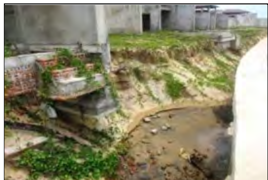
DIRECT DAMAGES OF EROSION
