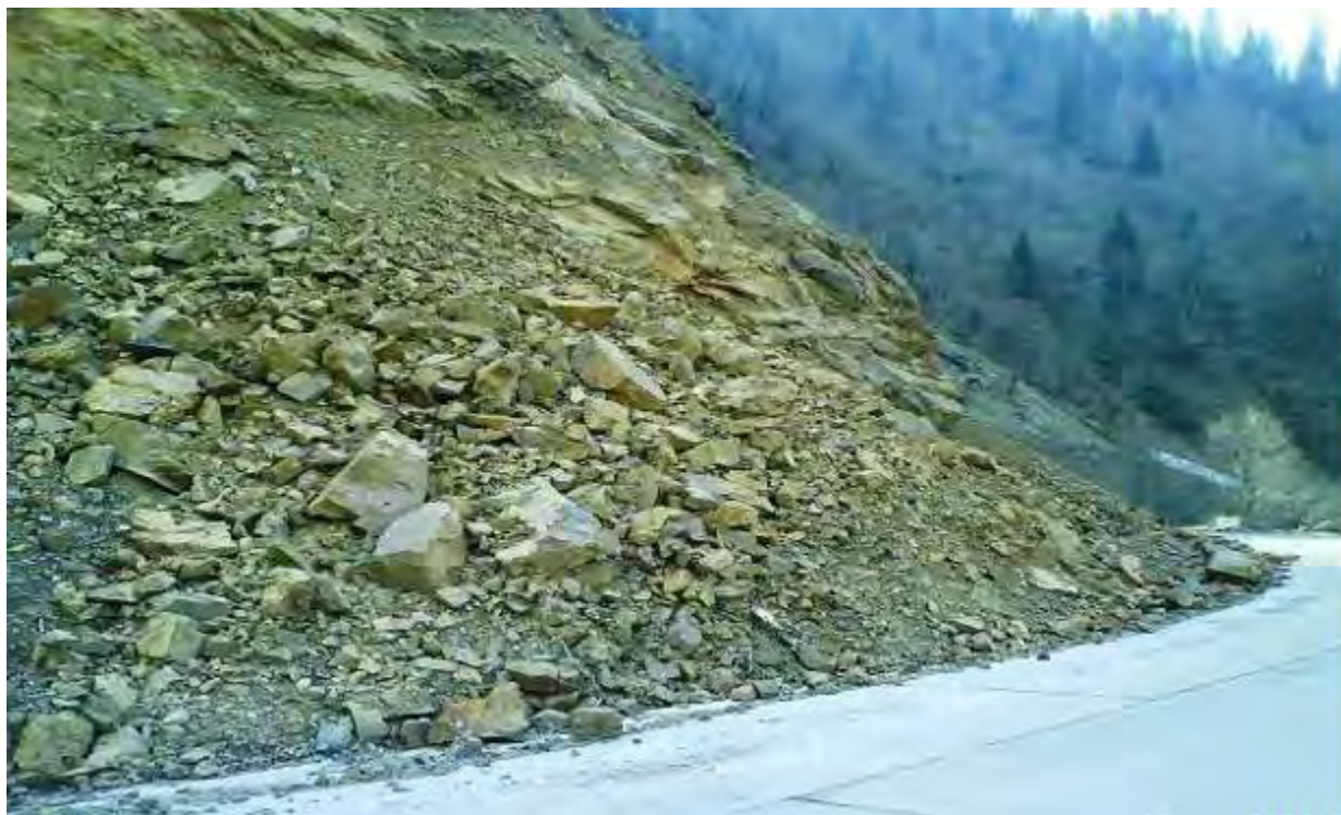
Figure 11. Material acumulated at the foot of the exposed slopes
