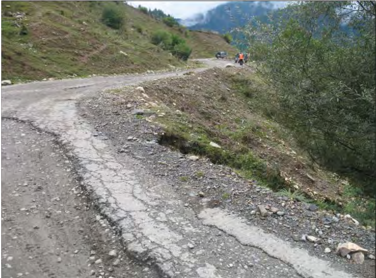
Figure 2. Asphalt-concrete and sand and gravel pavements at the I section of the project raud. Km 106
