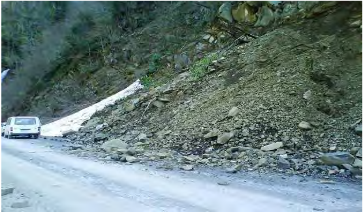
Figure 12. Material accumulated at the foot of the exposed slopes
