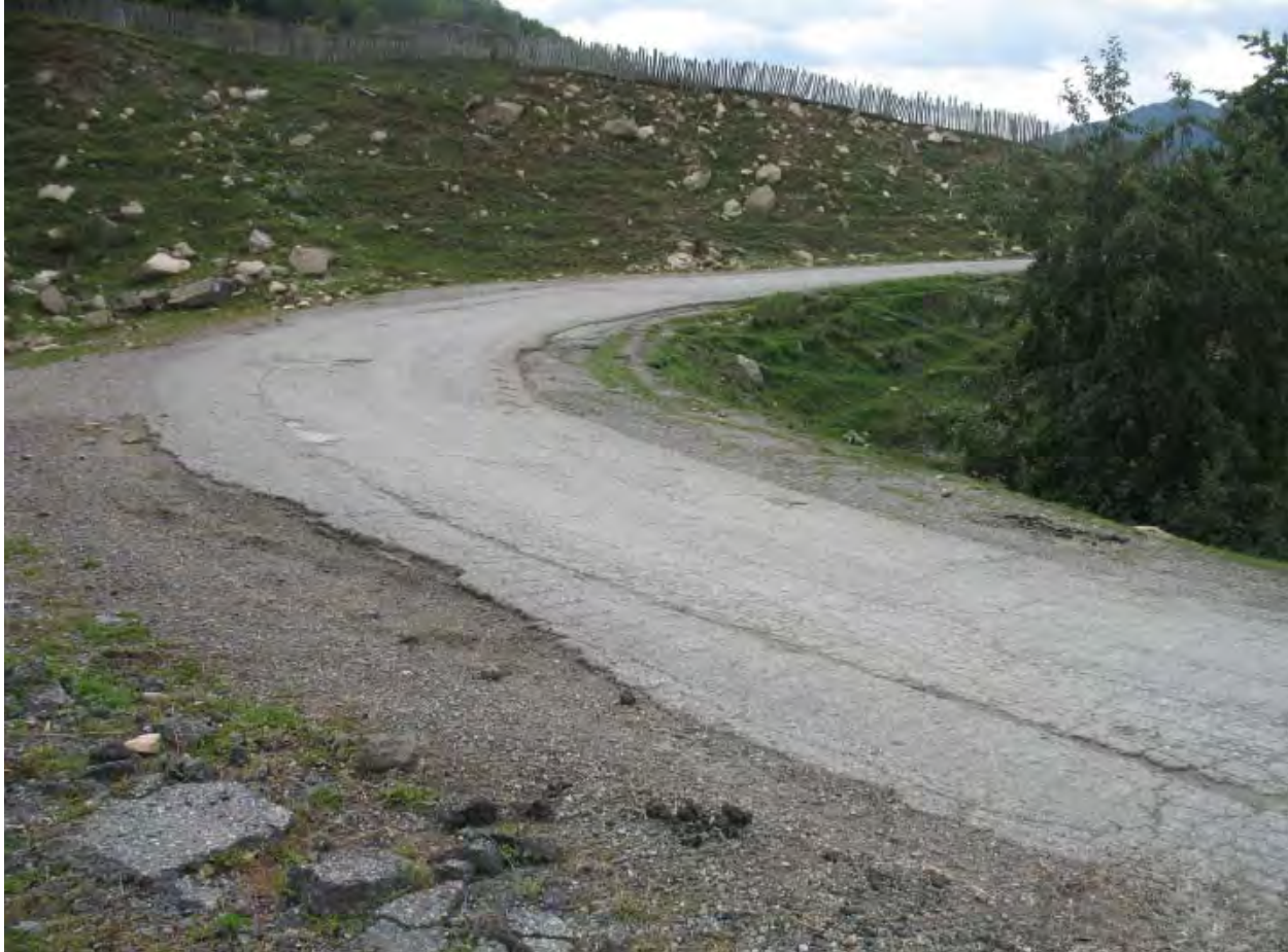
Figure 3. Asphalt-concrete and sand and gravel pavements at the II section of the project road. Km 113
