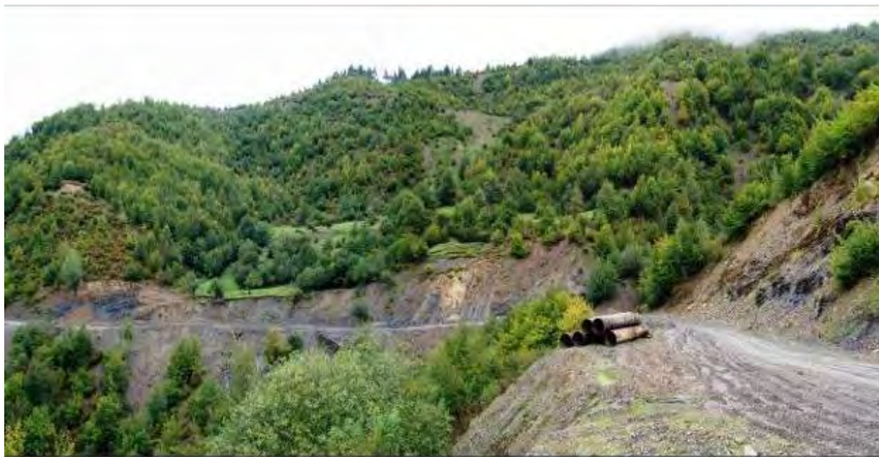
Figure 5. Landslide „Malatvibra” (114 Km)
