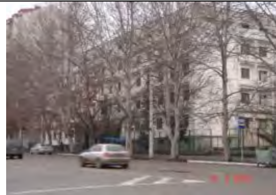
Fig.4.16: Medical center at Vaja Pshavela Ave
