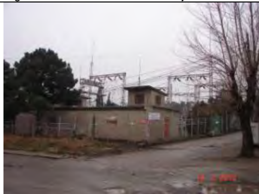
Fig.4.17: Power supply substation at Jikia St
