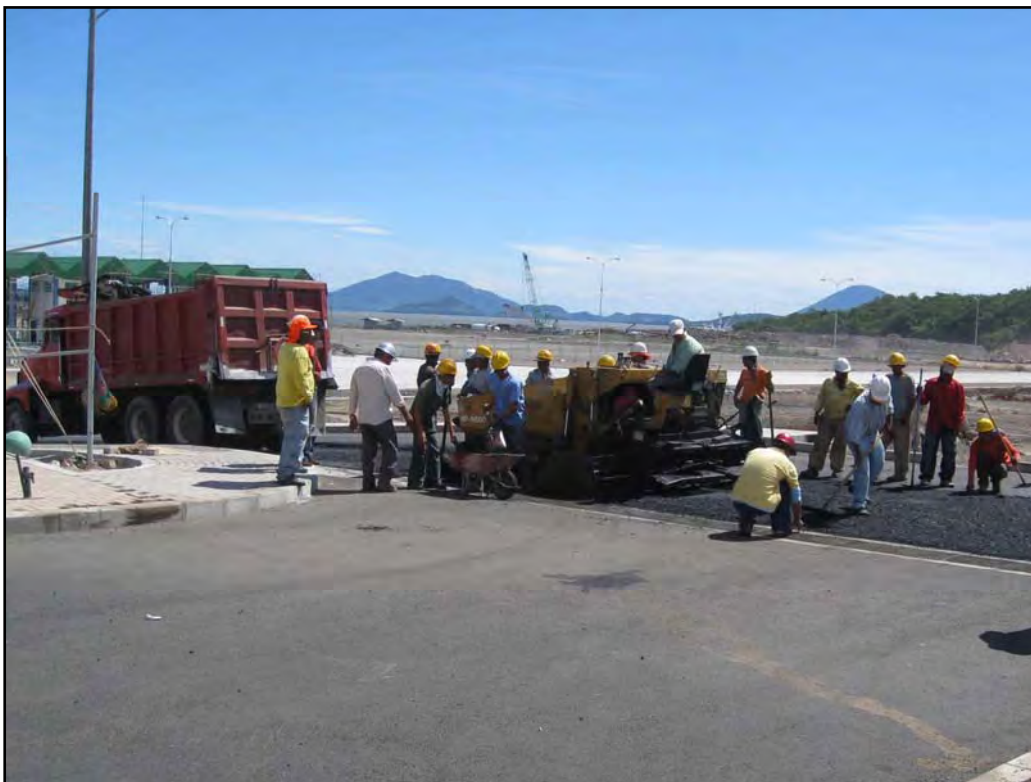
Photo 2: Team constructing a road using a small asphalting machine
