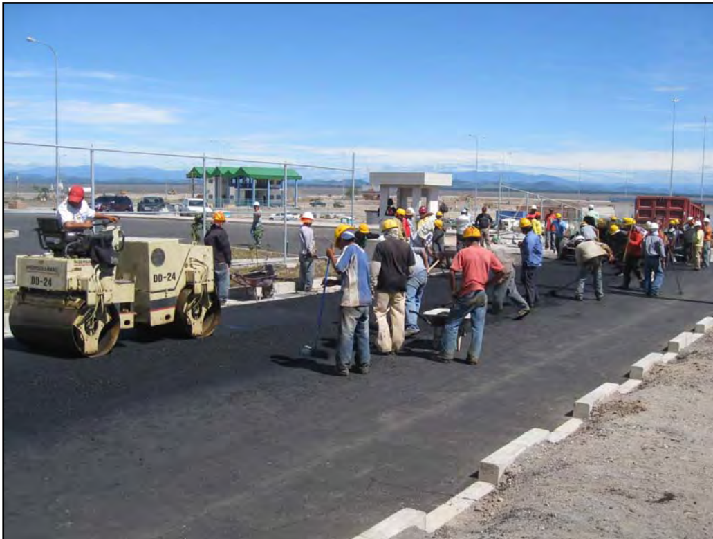
Photo 4: Roller vehicle being used in road construction
