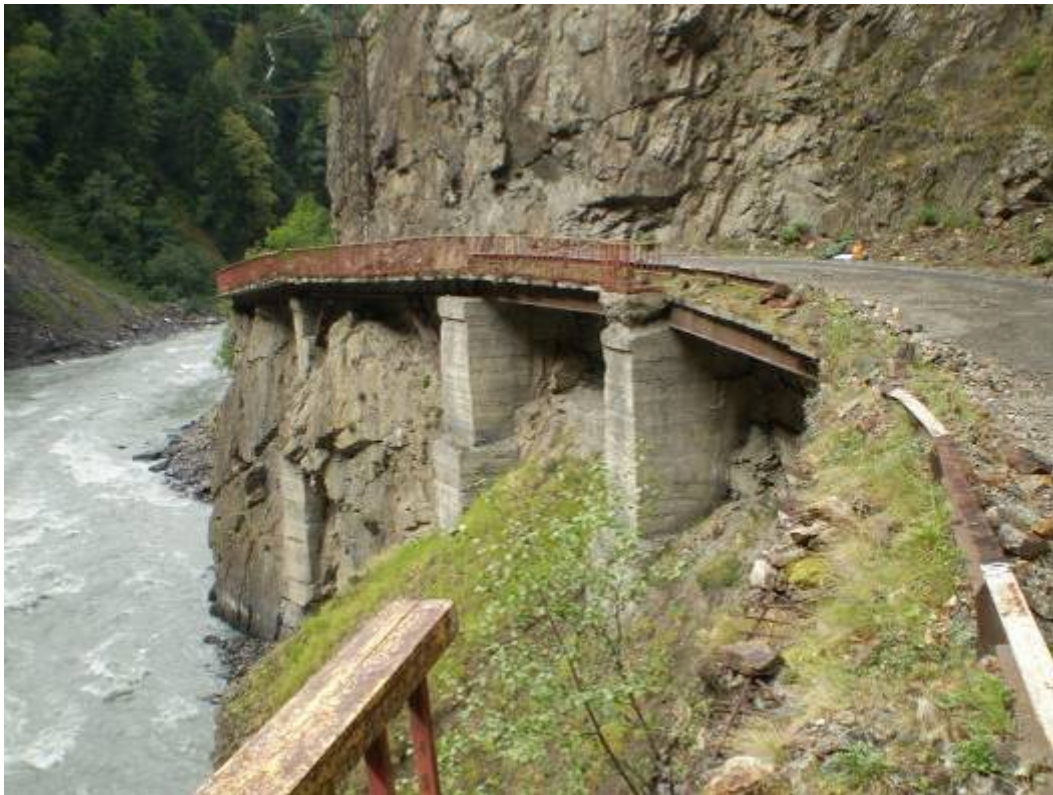
Fig.2 Existing Balcony on KM 89
