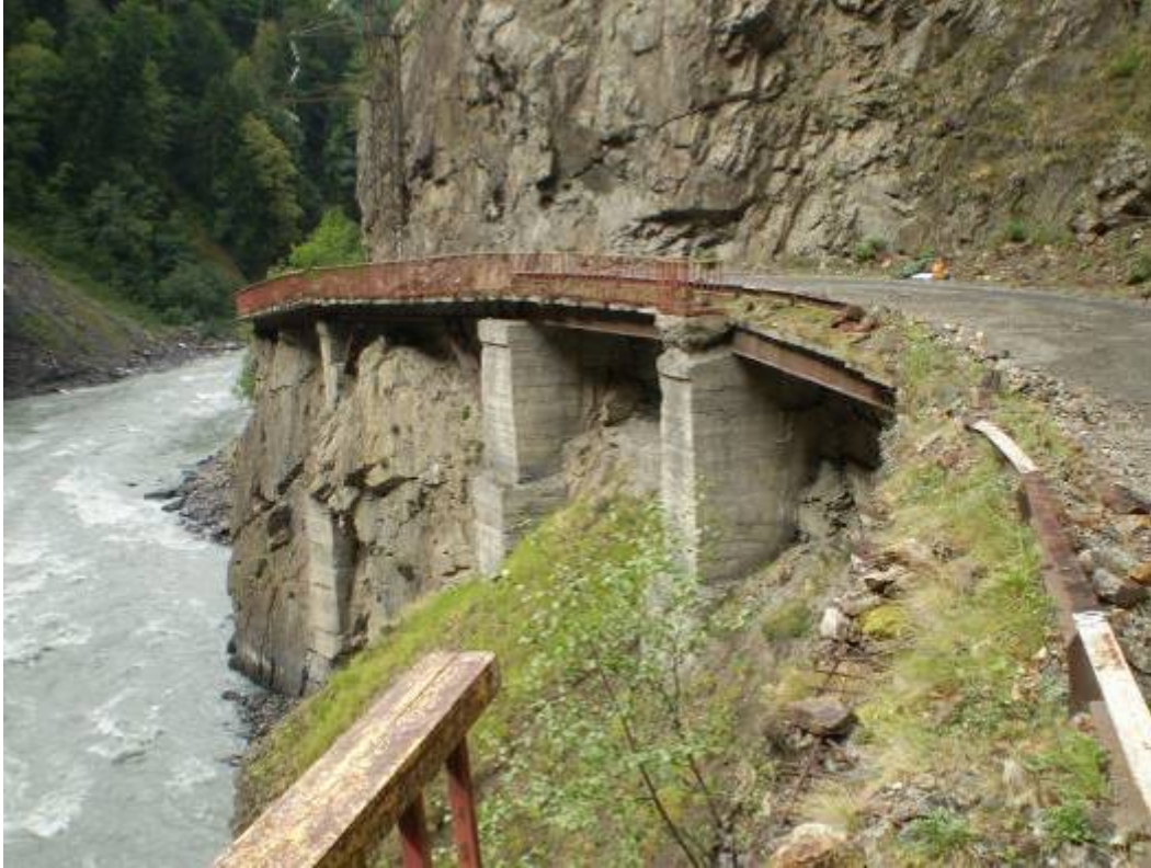
Fig.6. Existing Balcony located on km 89
