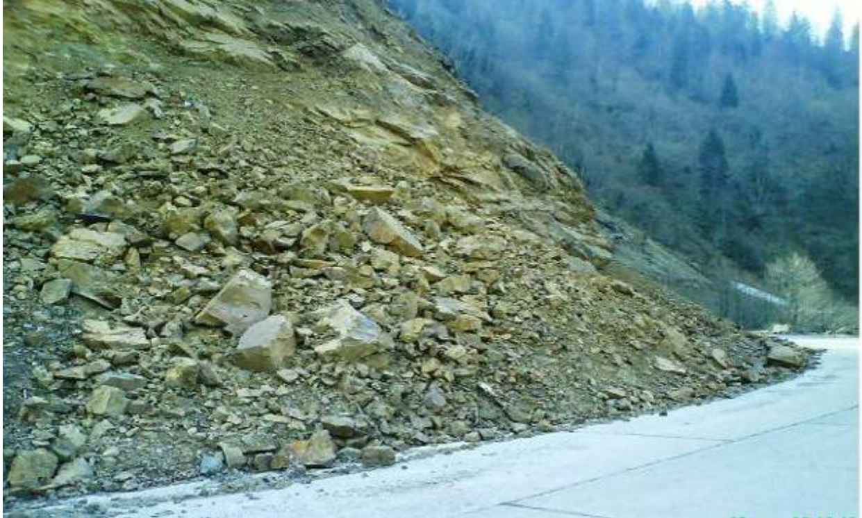
Figure 7. Material acumulated at the foot of the exposed slopes
