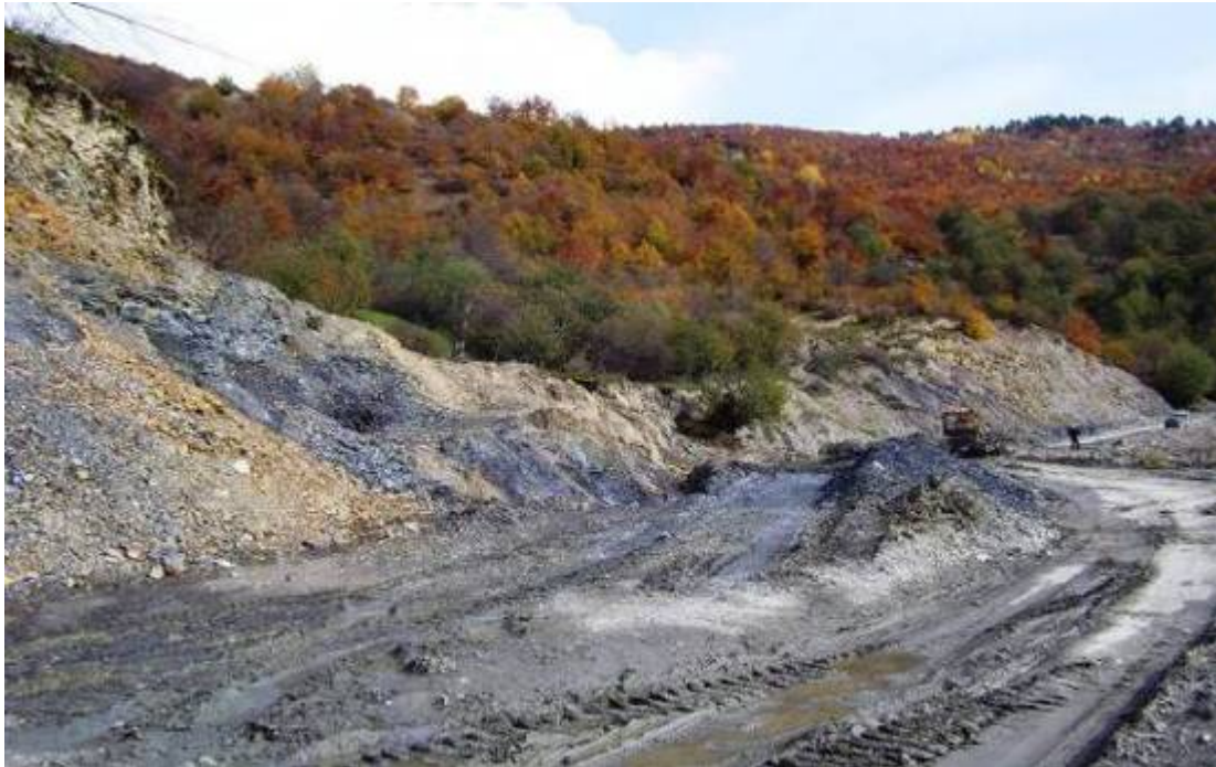
Fig10. Landslide “Malatvibra” (114 km)
