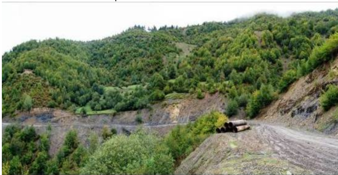
Fig 9. Landslide "Malatvibra" (114 km)
