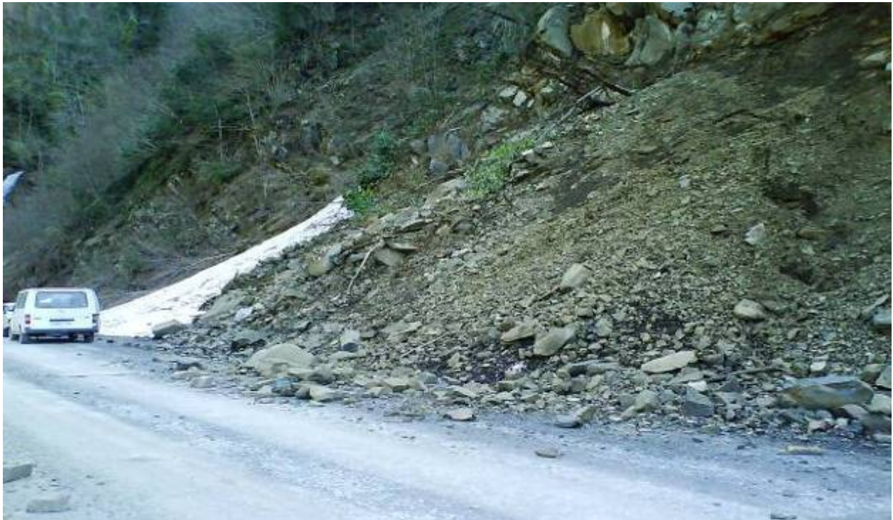
Figure 8. Material acumulated at the foot of the exposed slopes
