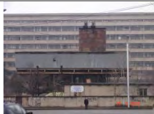
Fig.4.14 Shaft No.51 construction site
