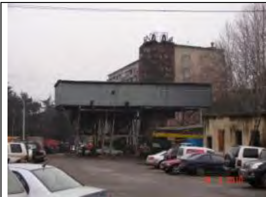
Fig.4.13 Shaft No.50 construction site
