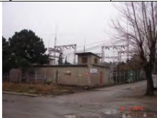
Fig.4.17: Power supply substation at Jikia St
