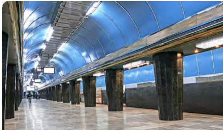
Fig. 4.10: Metro station Tsereteli
