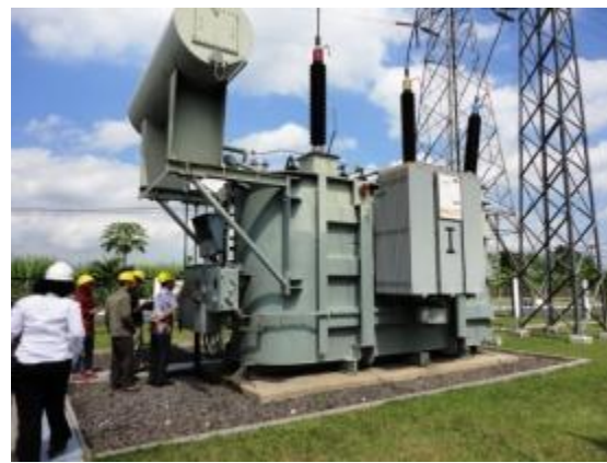
Figure 10. Existing 150/20 kVA, 30 MVA transformer at Tanggul – Jember.
