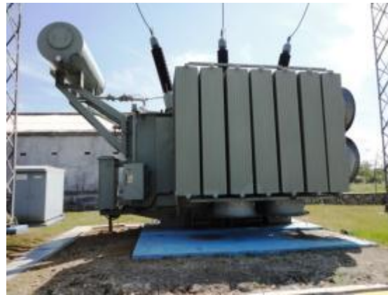
Figure 8. 150/20 kV 60MVA transformer at Sampang substation.
