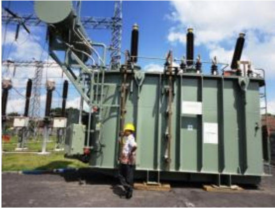
Figure 7. Typical new 150/20 kV 60 MVA transformer at Lumajang substation.
