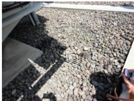
Figure 12. Oil spill containment berm at Tanggul Substation.
