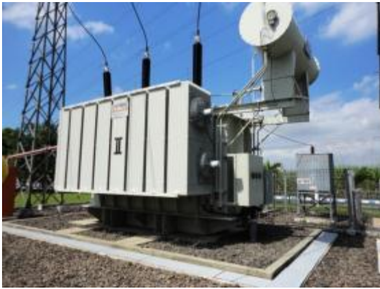
Figure 9. Existing 150/20 kVA 60MVA transformer at Tanggul – Jember.
