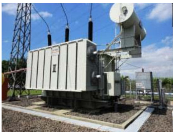
Figure 9. Existing 150/20 kVA 60MVA transformer at Tanggul – Jember.
