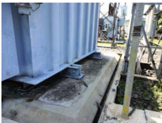
Figure 11. Oil spill containment berm. Oil will flow to an underground chamber in emergency situations. Negara substation – Bali.
