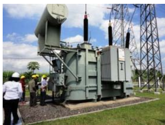
Figure 10. Existing 150/20 kVA, 30 MVA transformer at Tanggul – Jember.
