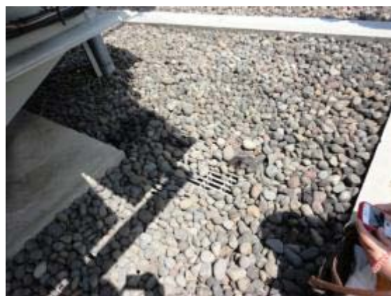
Figure 12. Oil spill containment berm at Tanggul Substation.
