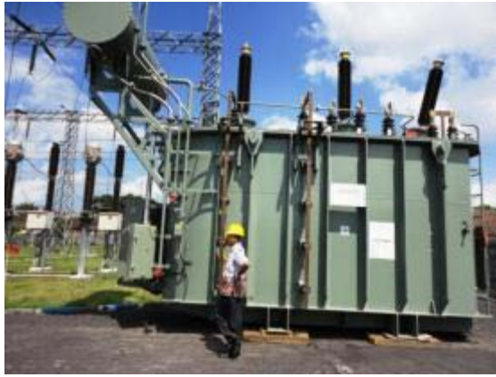
Figure 7. Typical new 150/20 kV 60 MVA transformer at Lumajang substation.
