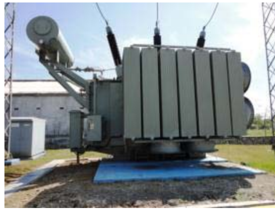
Figure 8. 150/20 kV 60MVA transformer at Sampang substation.
