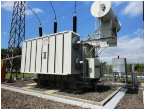
Figure 9. Existing 150/20 kVA 60MVA transformer at Tanggul – Jember.
