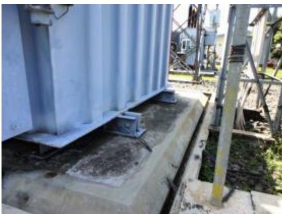
Figure 11. Oil spill containment berm. Oil will flow to an underground chamber in emergency situations. Negara substation – Bali.
