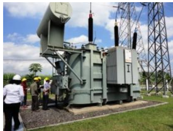
Figure 10. Existing 150/20 kVA, 30 MVA transformer at Tanggul – Jember.
