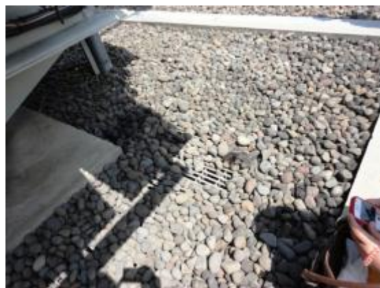
Figure 12. Oil spill containment berm at Tanggul Substation.
