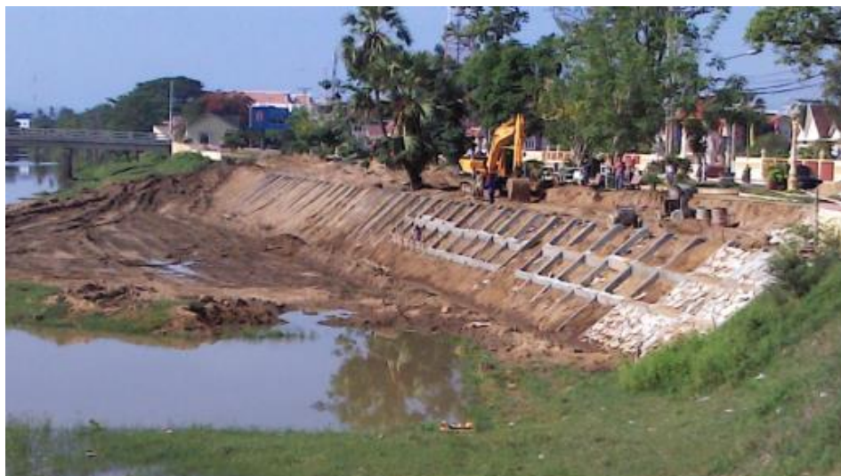
Figure B.8 Ongoing Embankment Protection Works in Pursat
