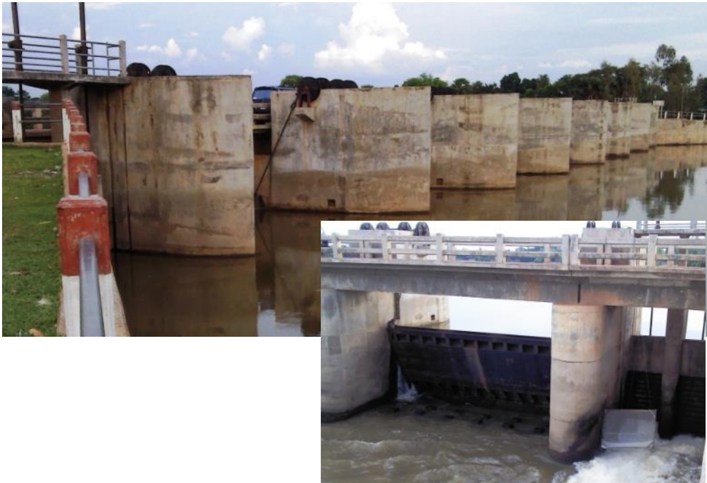
Figure B.3 Upstream Barrage on Pursat River with Flapgate Detail
