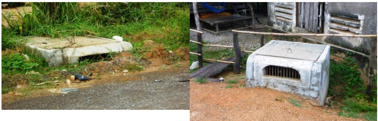
Figure B.7 Recently Constructed Drain Inlets
