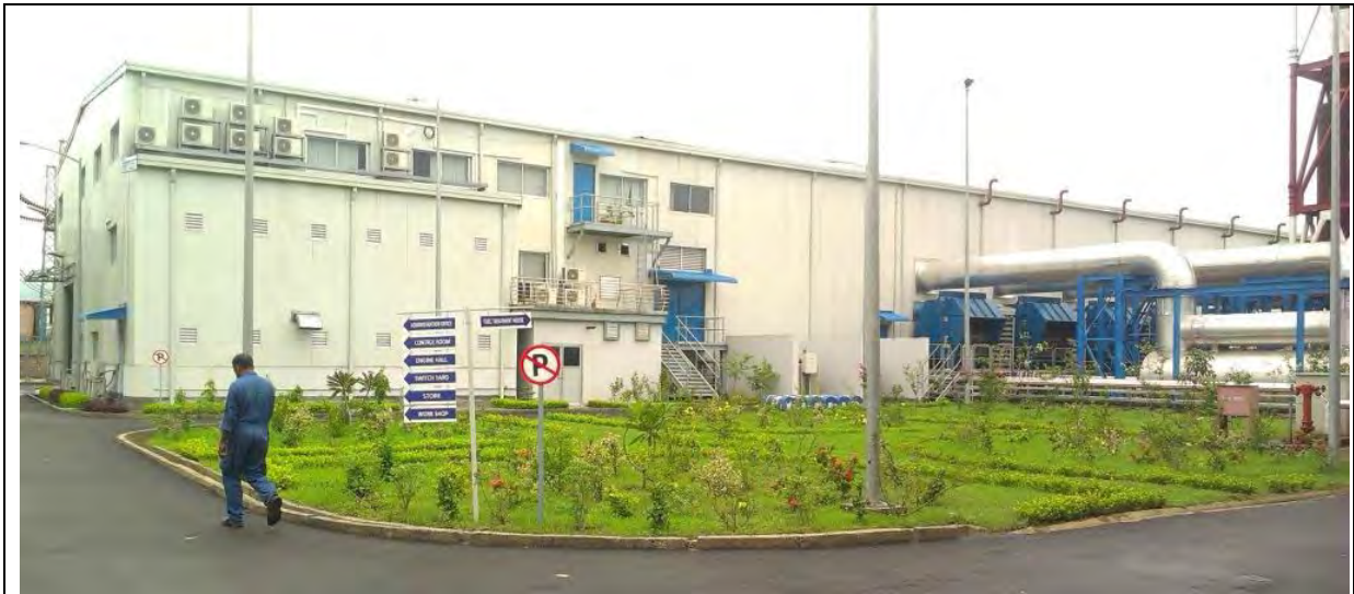
Photograph: External view of the plant (partial)
