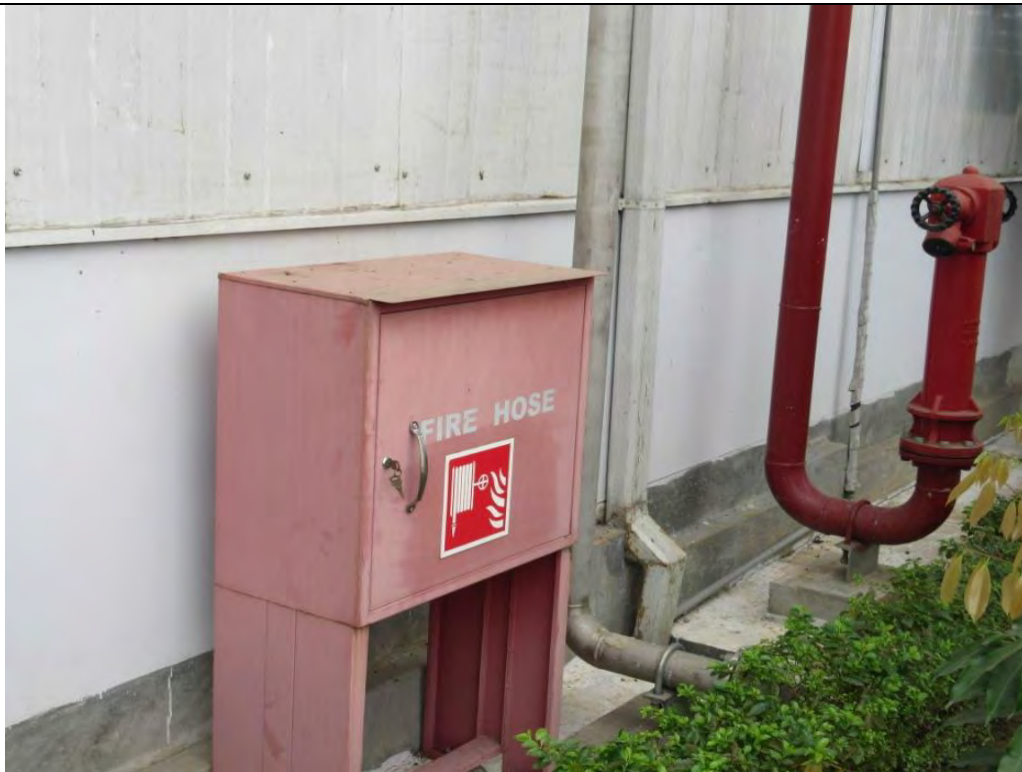
Photograph: Different types of fire-fighting arrangement
