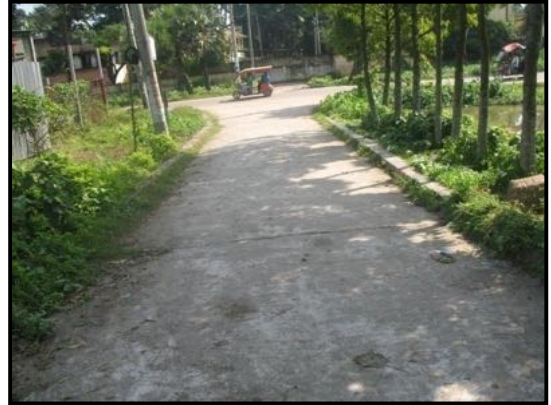
Photograph 3.3: An approach road to sub-station connecting site with Comilla-Laksham Road
