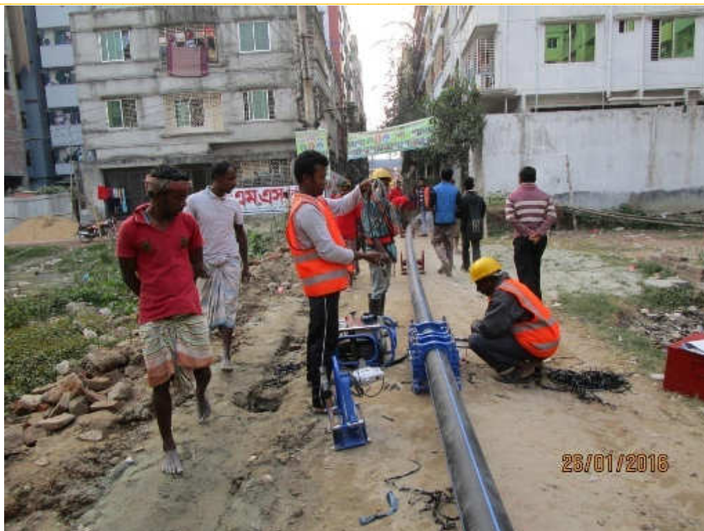
Photo 3: Pipe Jointing (Butt Fusion Method)
