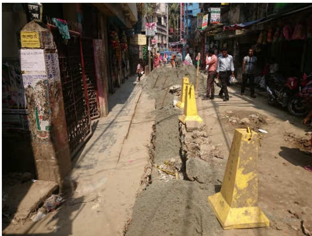
Photo 2: Backfilling of Trenches after Pipe Laying
