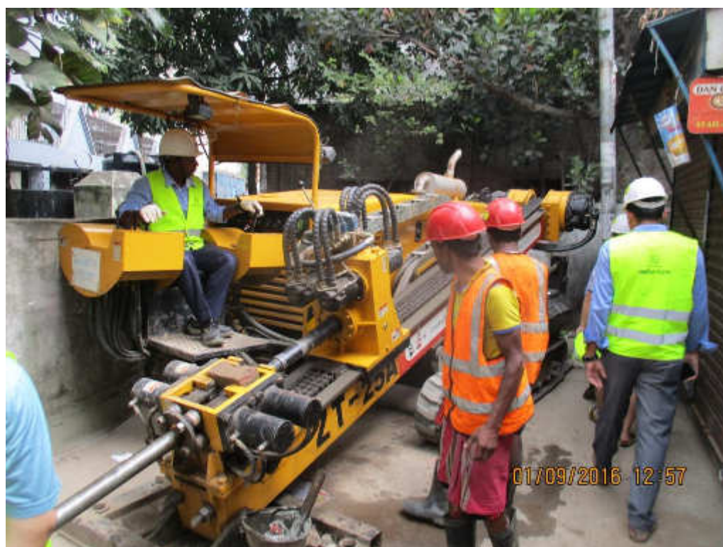
Photo 4: Horizontal Directional Drilling (HDD) Machine in Operation
