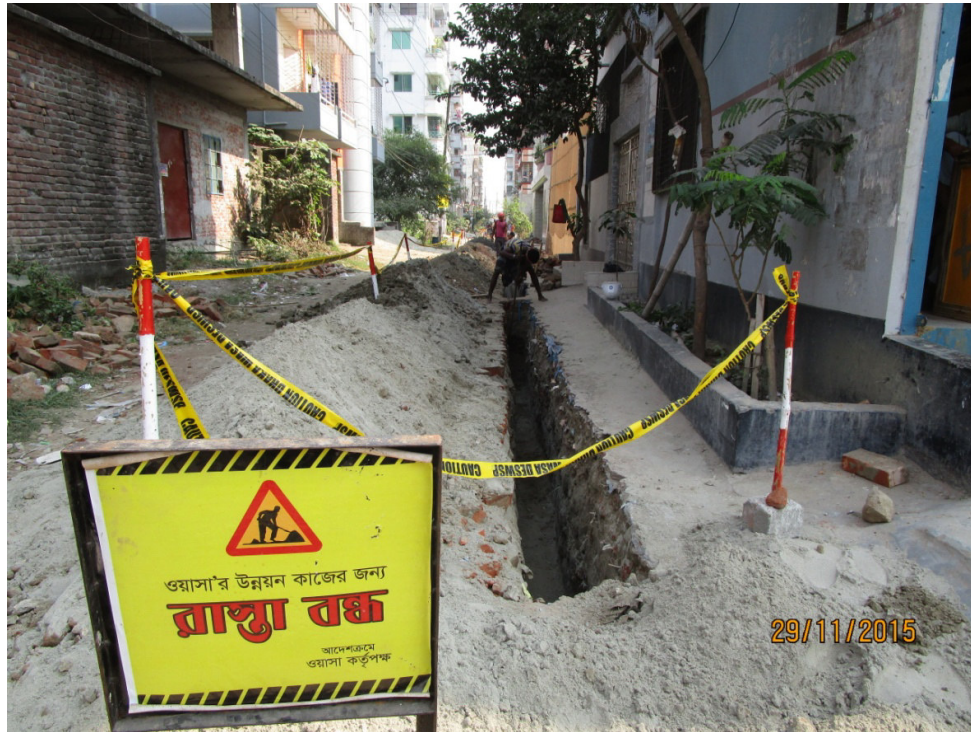
Fencing (plastic tape & bamboo posts) along the way of Open Trench
